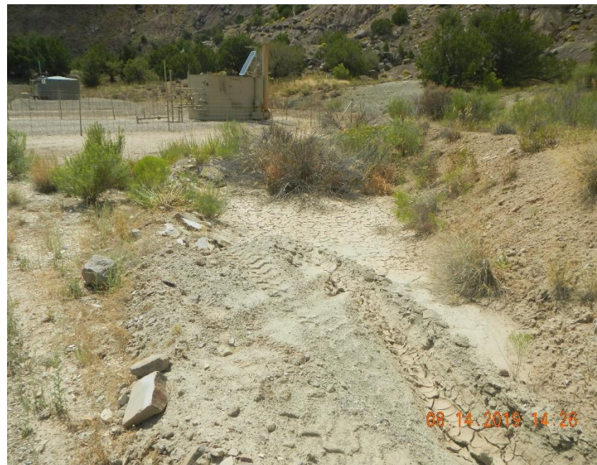
Sediment build up in checkdam at west side of entrance of location.
