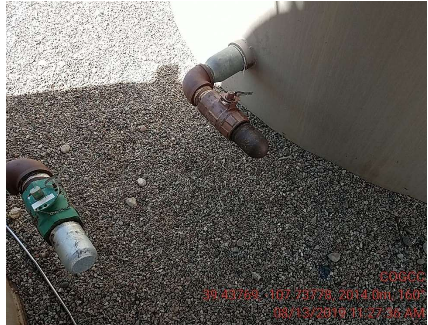
New photo of fixed valve and leak
