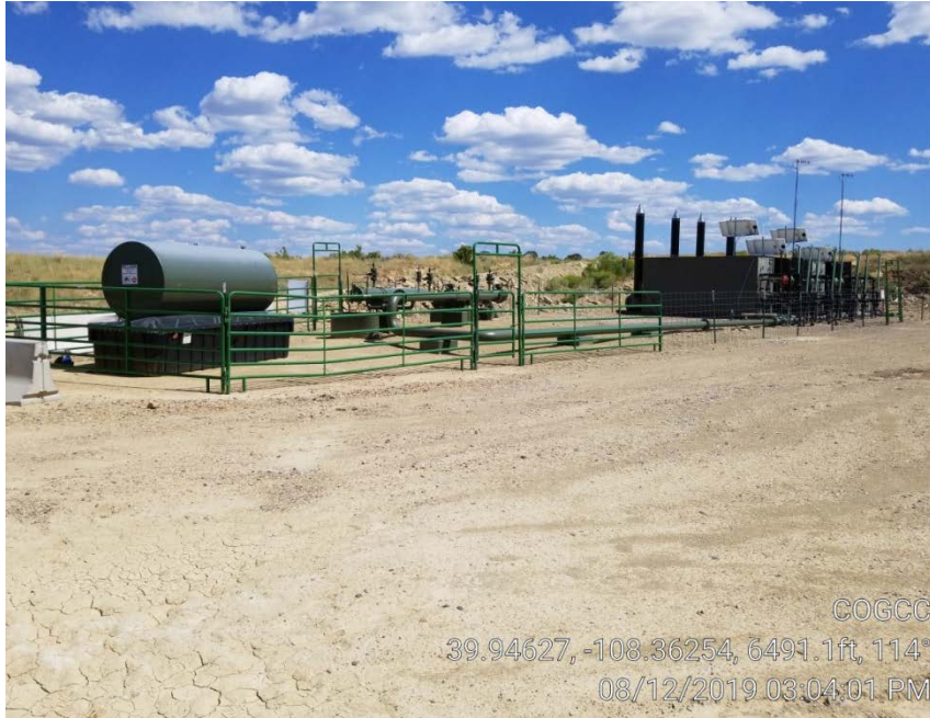
Photo 2. Separator & pig station.
