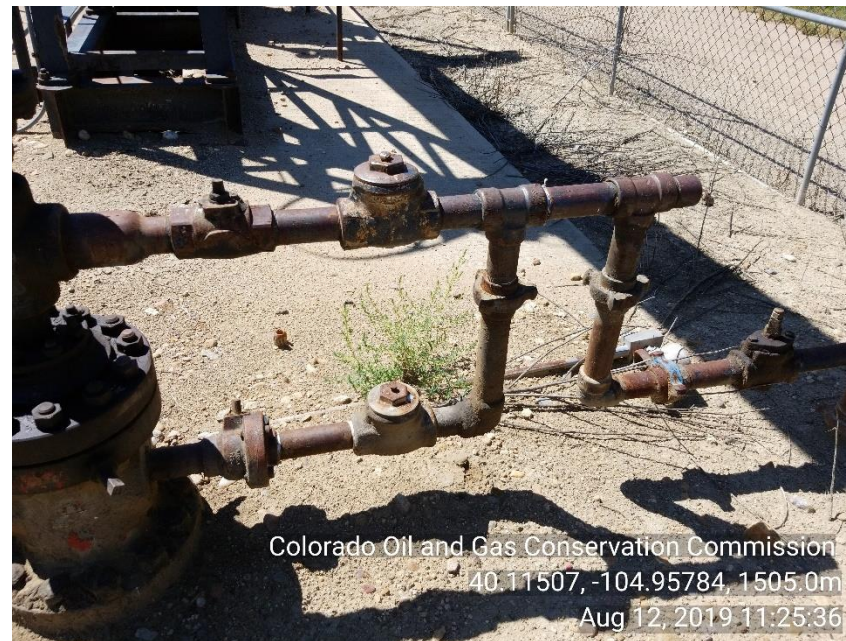
Photo 6 Production records show well as SI at time of inspection flow line valves are open and inspector can hear what appears to be gas flowing through flow lines.
