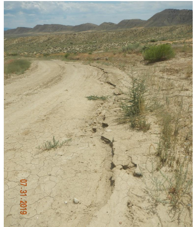
Photo#6: Erosion is occurring on both sides of access road
