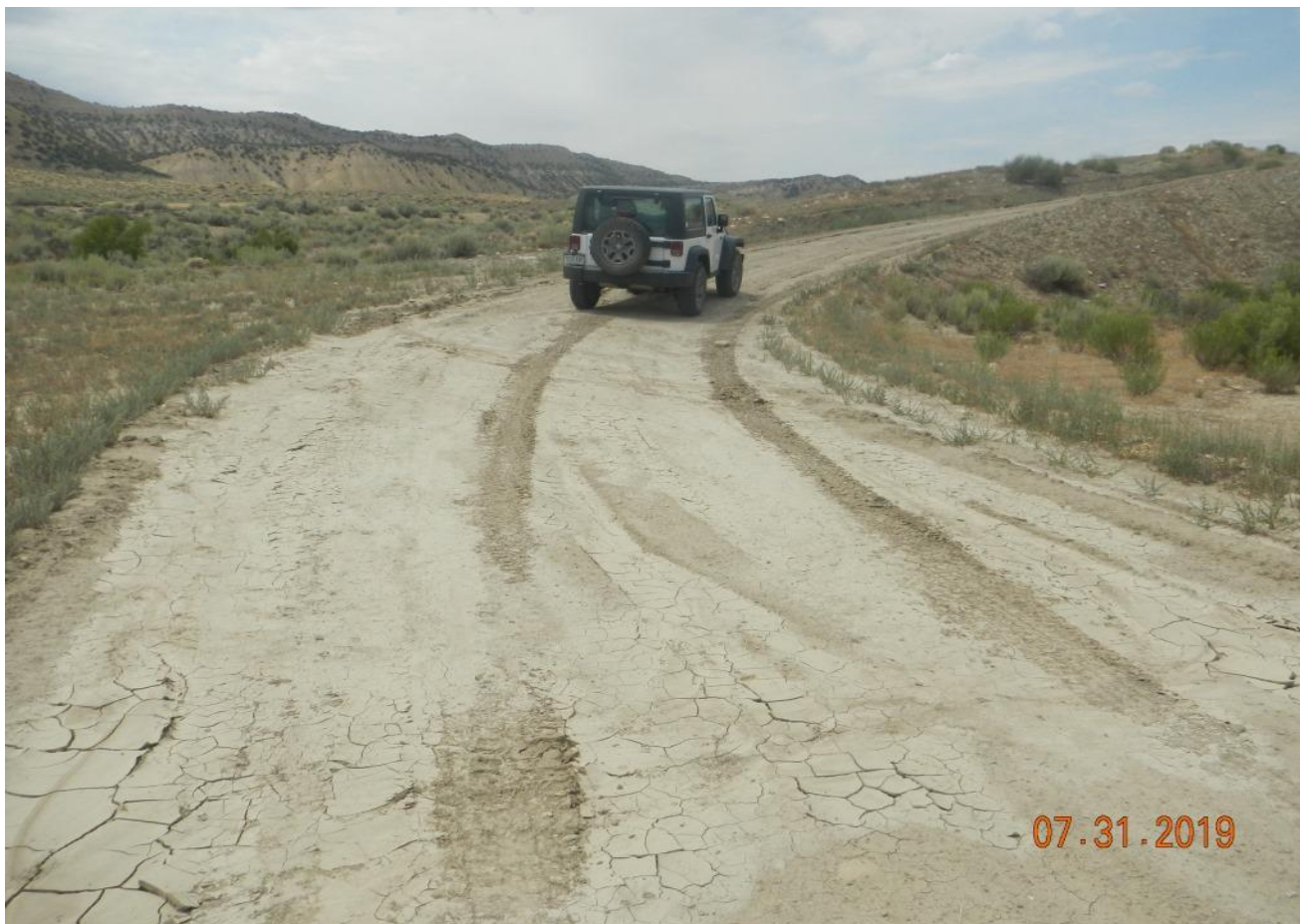
Photo#4: Sediment is collecting and migrating at base of Access Road.
