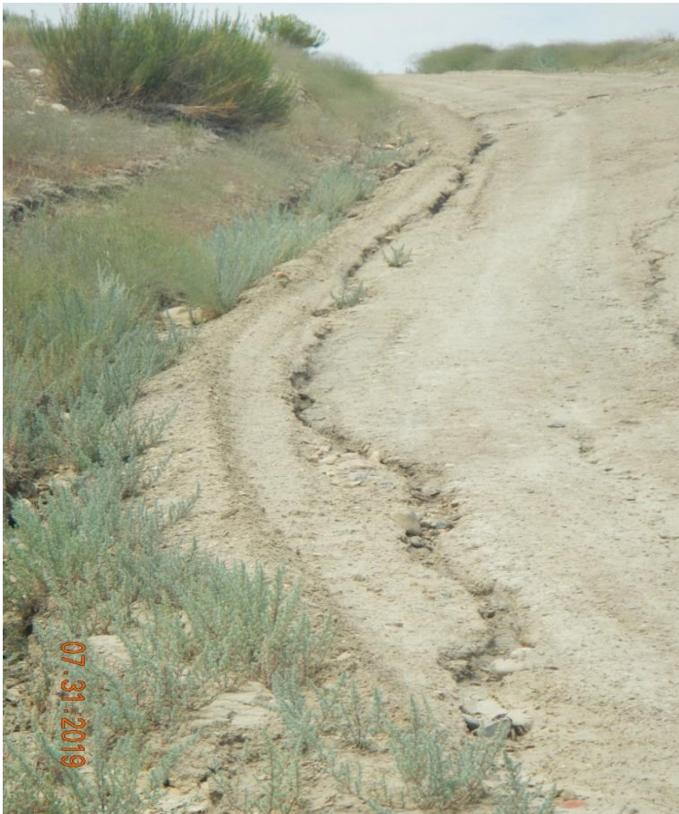
Photo#5: Erosion is occurring on both sides of access road.
