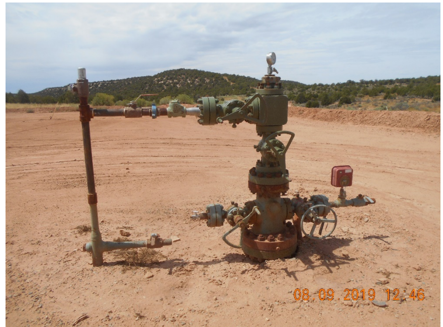
Injection wellhead..
