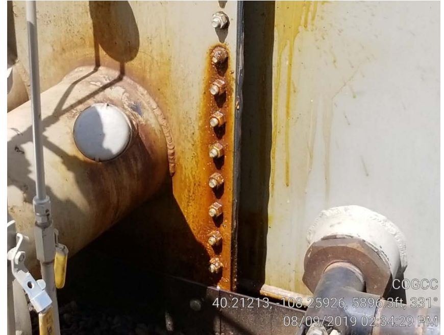
Photo 5. 500 bbl tank leaking oil.
