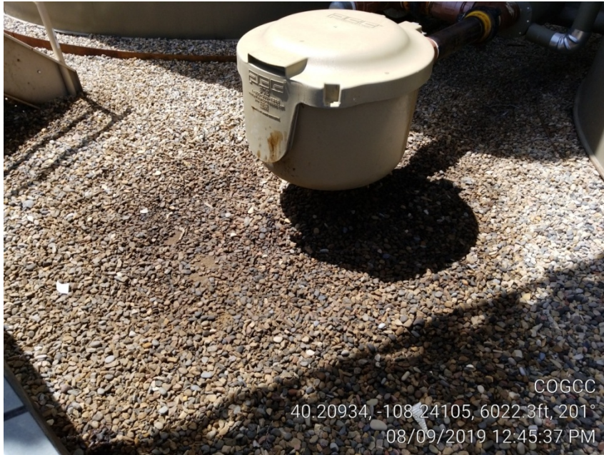
Photo 6. Stained gravel next to oil tank valve.
