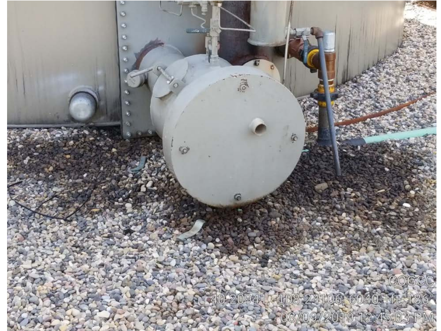
Photo 5. Stained gravel at base of tubing next to tank burner.
