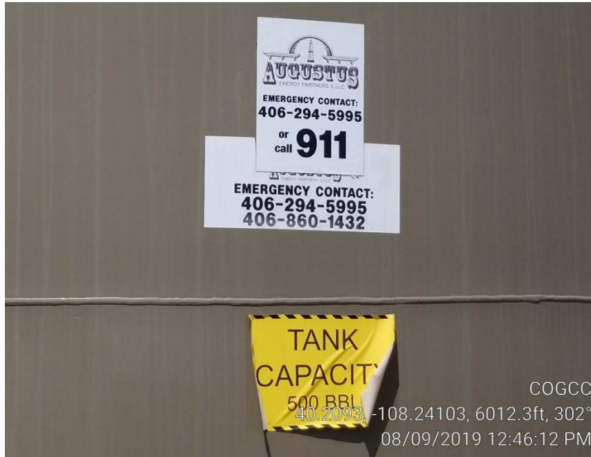
Photo 8. Tank missing contents & NFPA label.
