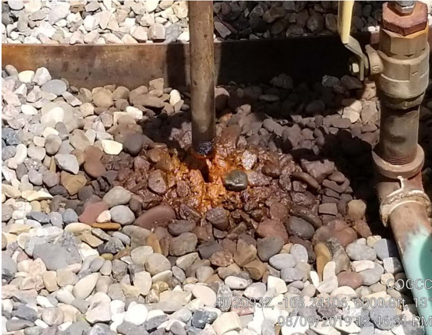
Photo 4. Stained gravel at base of tubing next to tank burner.
