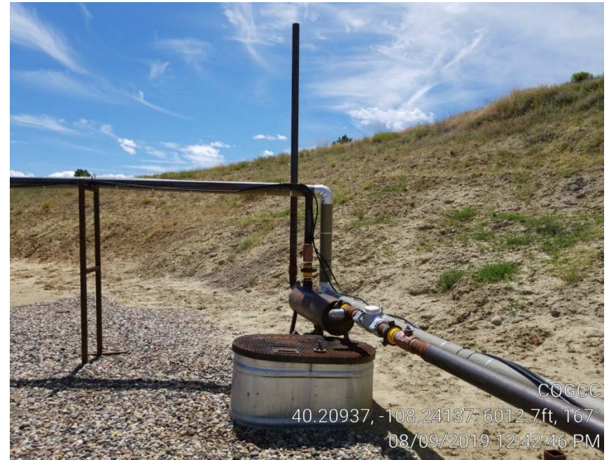
Photo 13. Vent without bird protection.
