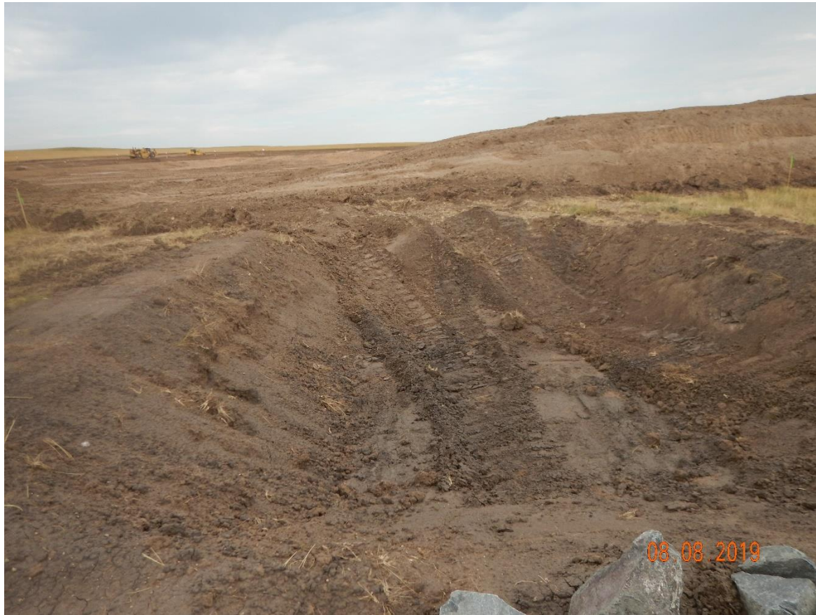
Photo 4: Photo taken of sediment trap. Sediment traps have not been constructed in accordance with good engineering practices; traps do not appear to be sufficient in size to manage runoff from the 10+ acre pad, berms/ slopes of traps remain unconsolidated. BMPs missing inlet armoring/protection. Rock aggregate used for outlet protection appears too large in size to slow stormwater discharge, trap sediment and sufficiently stabilize outlet.
