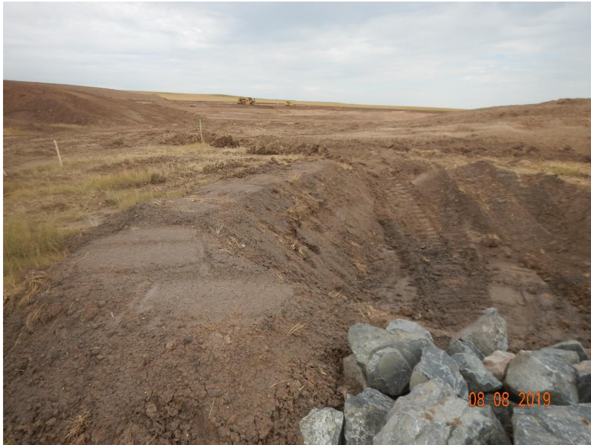
Photo 2: See comments under photo 1. Photo also shows one of the three stormwater sediment traps on the south end of the location. Sediment traps have not been constructed in accordance with good engineering practices; traps do not appear to be sufficient in size to manage runoff from the 10+ acre pad, berms at traps remain unconsolidated. BMPs missing inlet armoring/protection. Rock aggregate used for outlet protection appears too large in size to slow stormwater discharge, trap sediment and sufficiently stabilize outlet.
