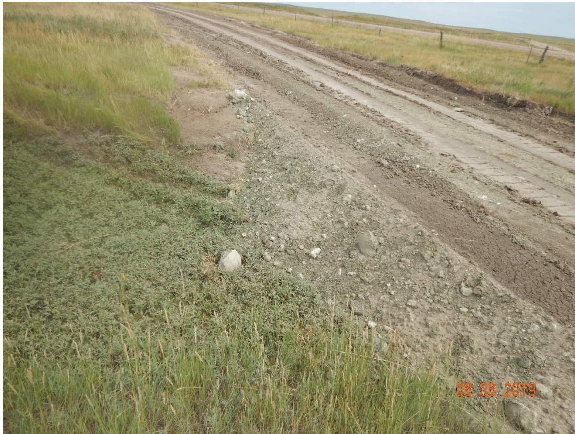
Photo 8: Photo taken from the access road, facing north. Photo shows area of access road that was constructed across a drainage. No BMPs have been installed to prevent ponding and allow for water movement under access road. Additionally no tracking BMPs have been installed to mitigate sediment transport off location.
