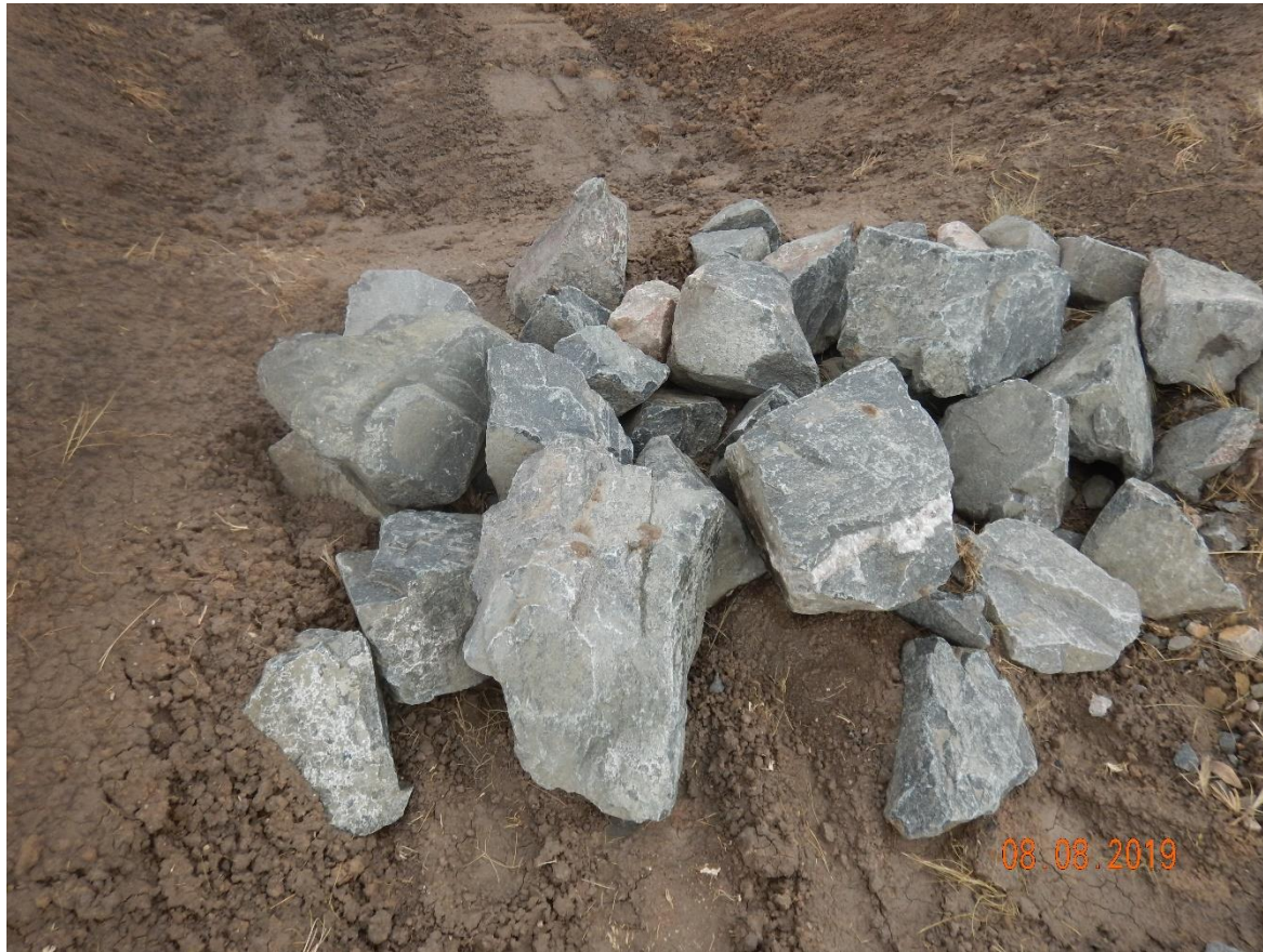
Photo 3: Photo of rock aggregate used at the sediment trap outlet. Rock aggregate used for outlet protection appears too large in size to slow stormwater discharge, trap sediment and sufficiently stabilize outlet.
