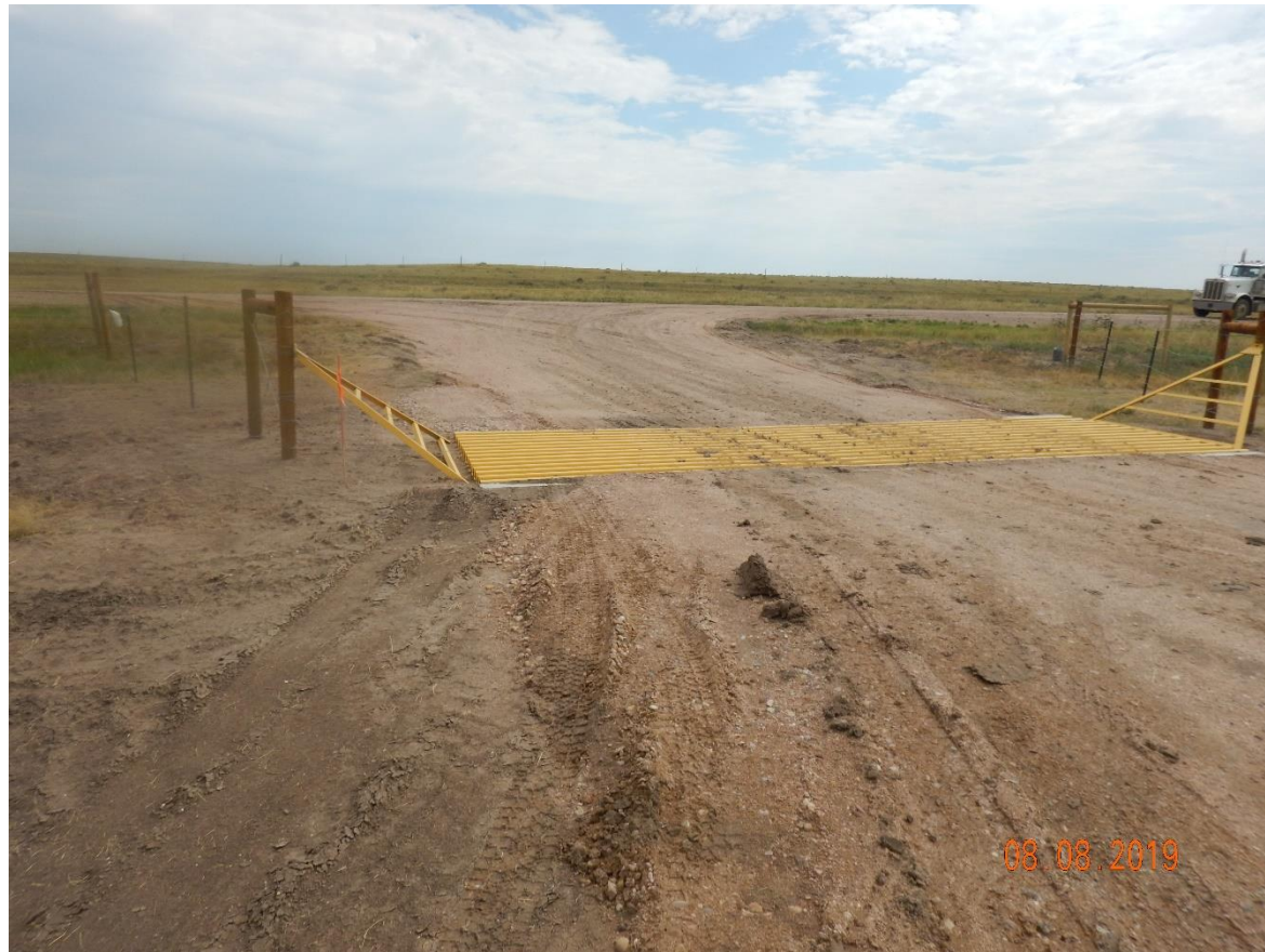
Photo 9: Photo taken from the access road entrance, facing east. Photo shows no tracking BMPs have been installed to mitigate sediment transport off location.
