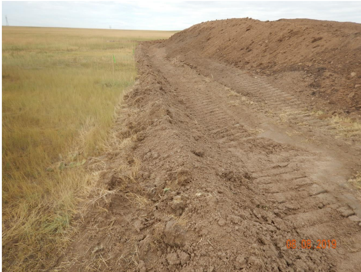
Photo 5: Photo taken from the south end of the location, facing west. Operator has removed surface roughening and installed a stormwater ditch/berm along the perimeter of the pad. Ditch/berm has not been installed in accordance with good engineering practices; Ditch/berm remains loose, unconsolidated material. Ditch appears to have been cut with a single pass of a blade, and has been left with a steep grade on one side that can result in stormwater incision within the ditch.
