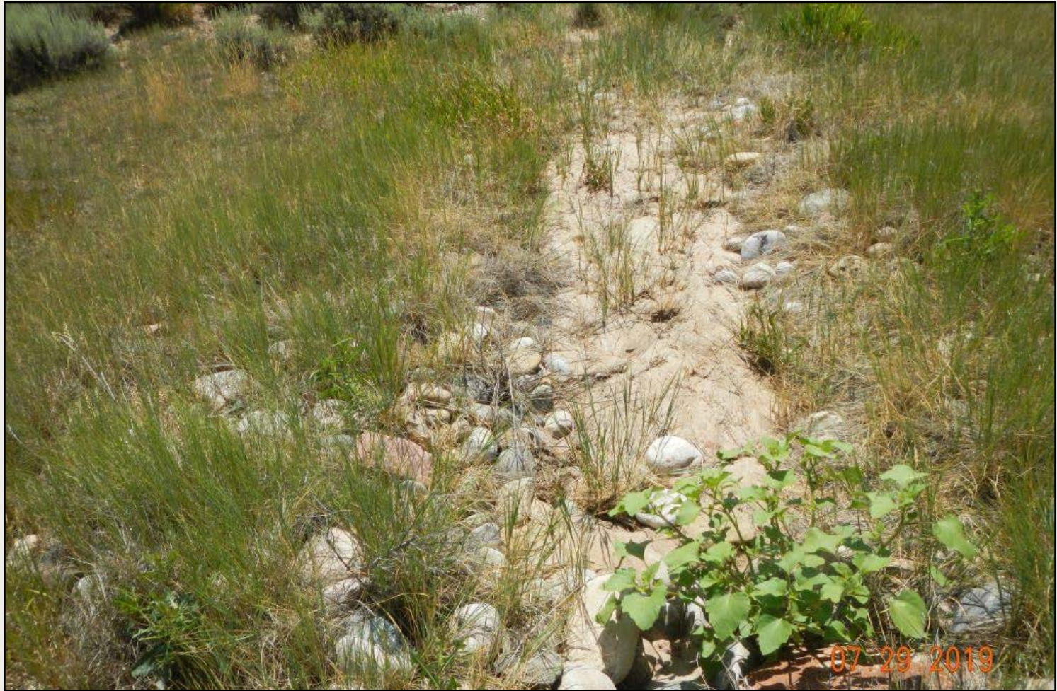
Photo 5. View of sediment-filled channel at culvert outlet along the access road.
