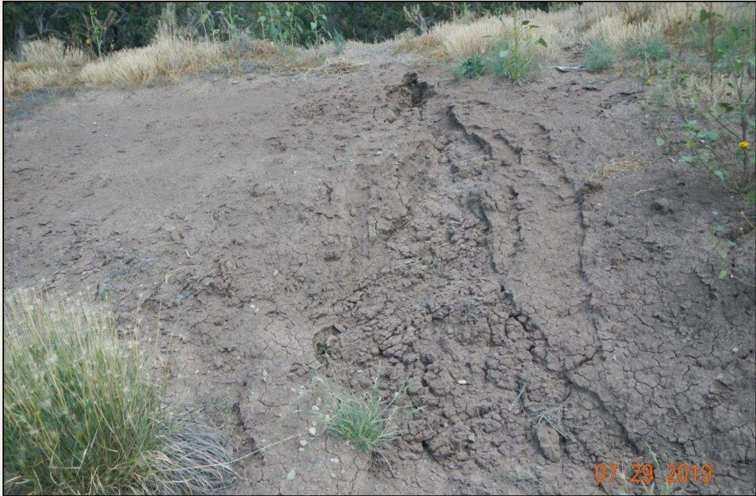
Photo 4. View of erosional channel within the northern cut-slope.
