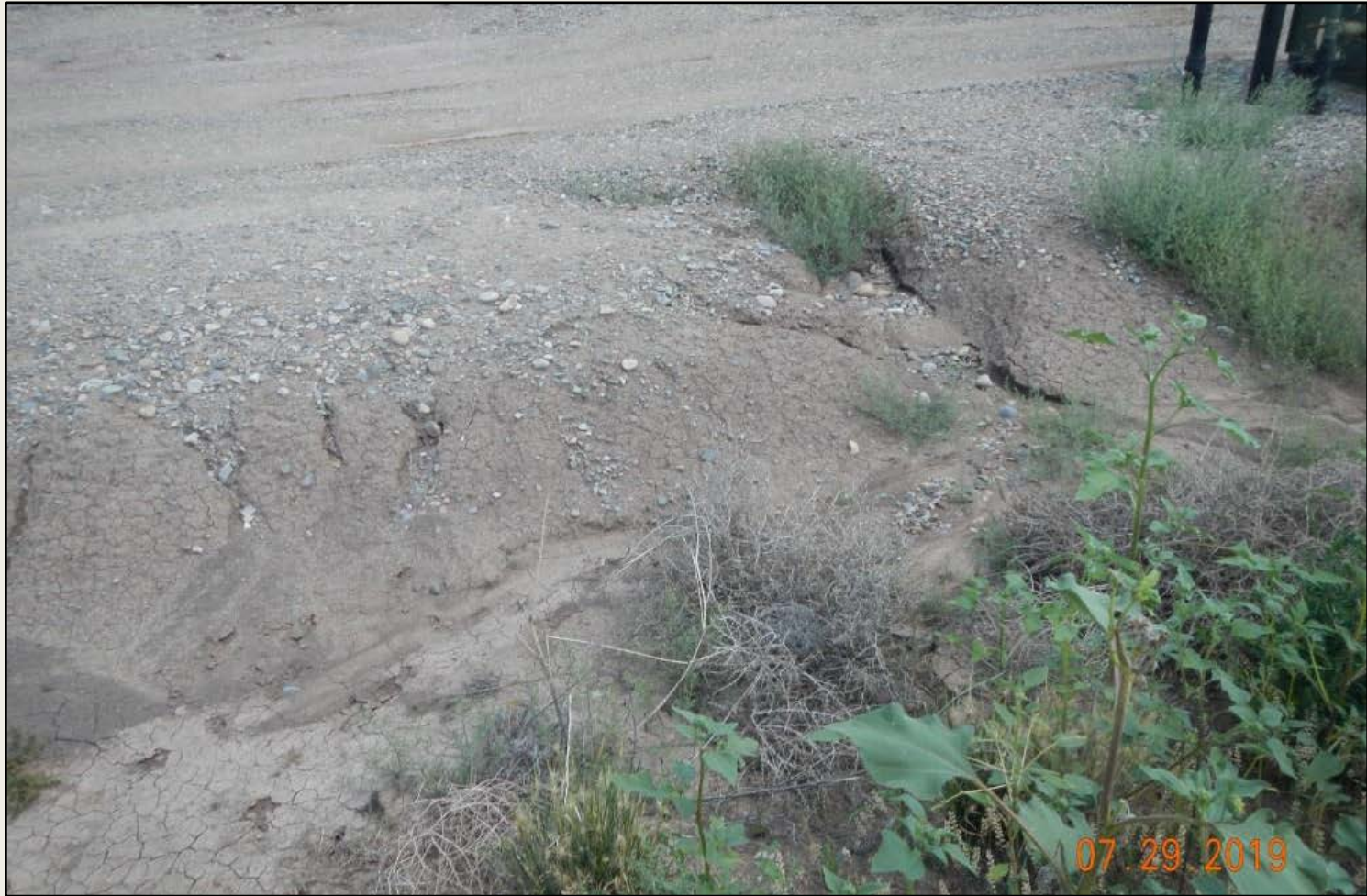
Photo 1. View of erosional channeling and sedimentation along the southern edge of the well pad.
