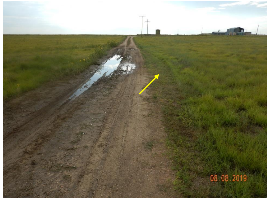
Photo 4: Photo taken from the access road, facing east. Photo shows operator has travelled beyond the designated access road onto adjacent lands. This does not comply with 1002.e. Access road will need to be constructed with sufficient BMPs to allow for proper stormwater discharge to ensure existing access road remains in proper functioning condition.
