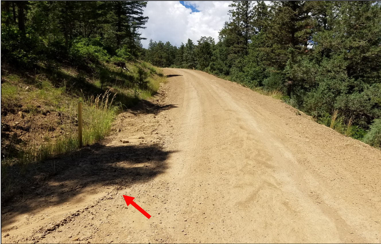
Photo 2. Vehicle ruts have been graded out, however it appears stormwater is not being directed toward the culvert. A little shovel work can fix this issue before it becomes bigger. Lat/Long:37.08032/-104.93209
