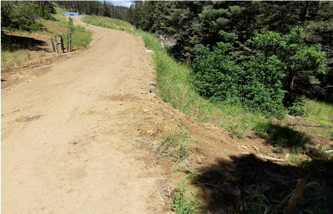
Photo 1. The culvert was cleaned out along the road. Material put on the road contains large rocks.
