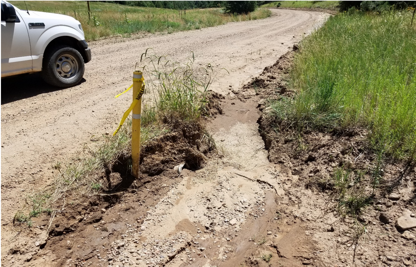
Photo 1. The culvert has filled in with sediment along the main road.
