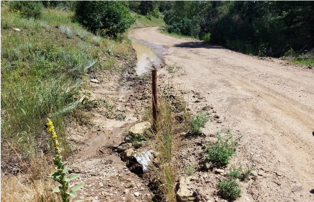
Photo 3. The culvert has filled in with sediment along the main road. Different culvert than previous photo.
