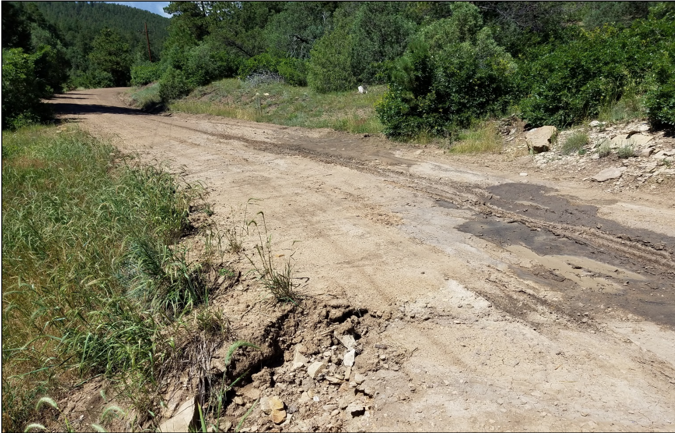
Photo 4. Stormwater is flowing across the road at this point. Culvert is filled in with sediment. Different culvert than previous photo.
