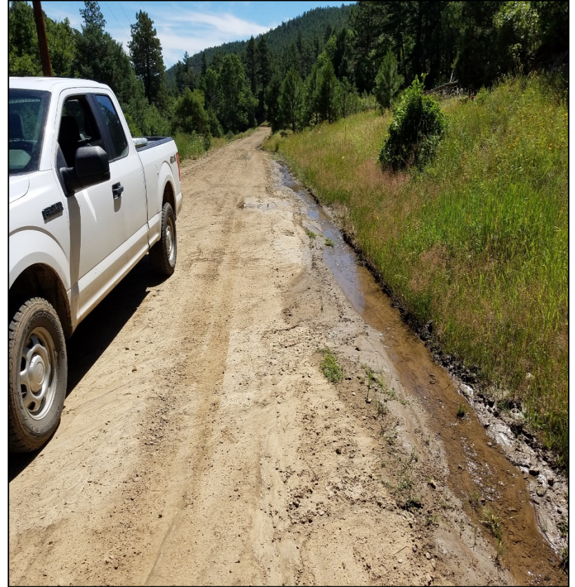
Photo 5. Water from the ephemeral creek is flowing down the side of the road. The culvert is filled in with sediment. Lat/Long: 37.089264/-104.954179
