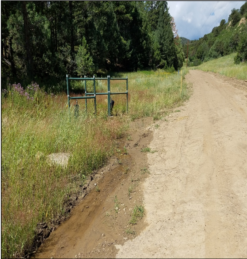
Photo 5. Water from the ephemeral creek is flowing down the side of the road. The culvert is filled in with sediment. Lat/Long: 37.089264/-104.954179
