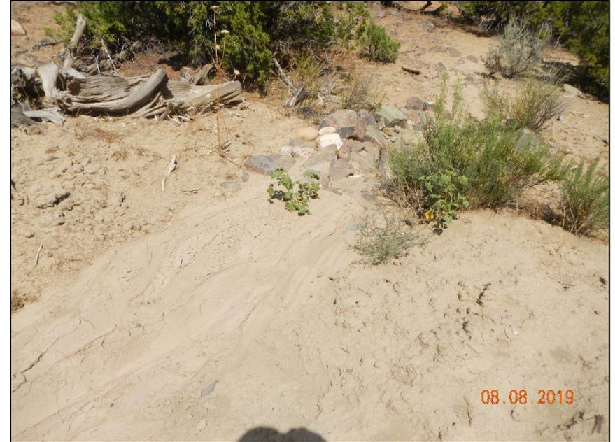
**Photo #8 Sediment traps on access road need maintenance**
