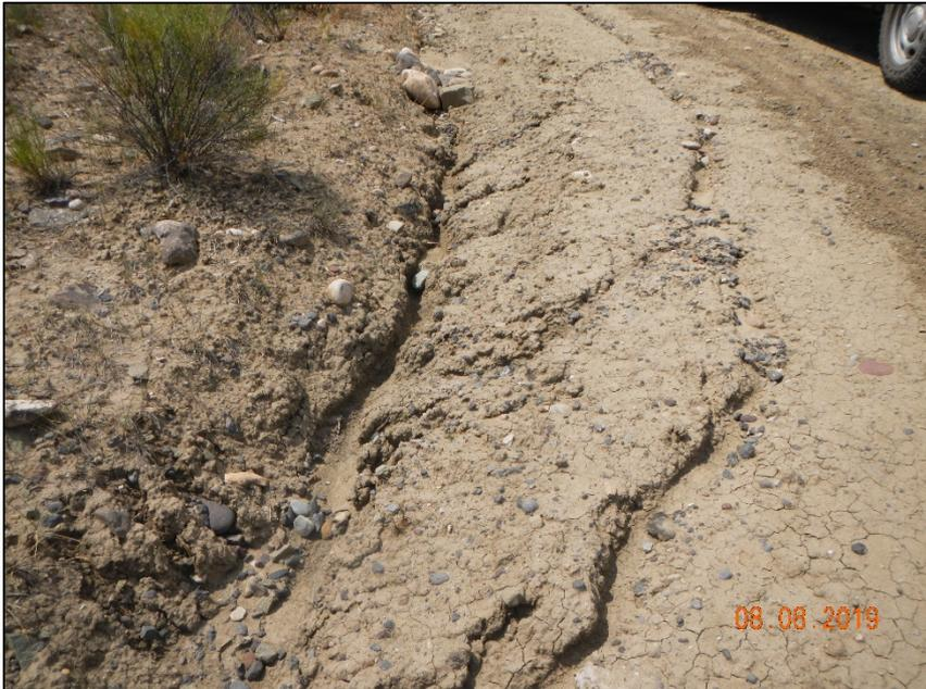
Photo #10 Check dams on access road need maintenance
