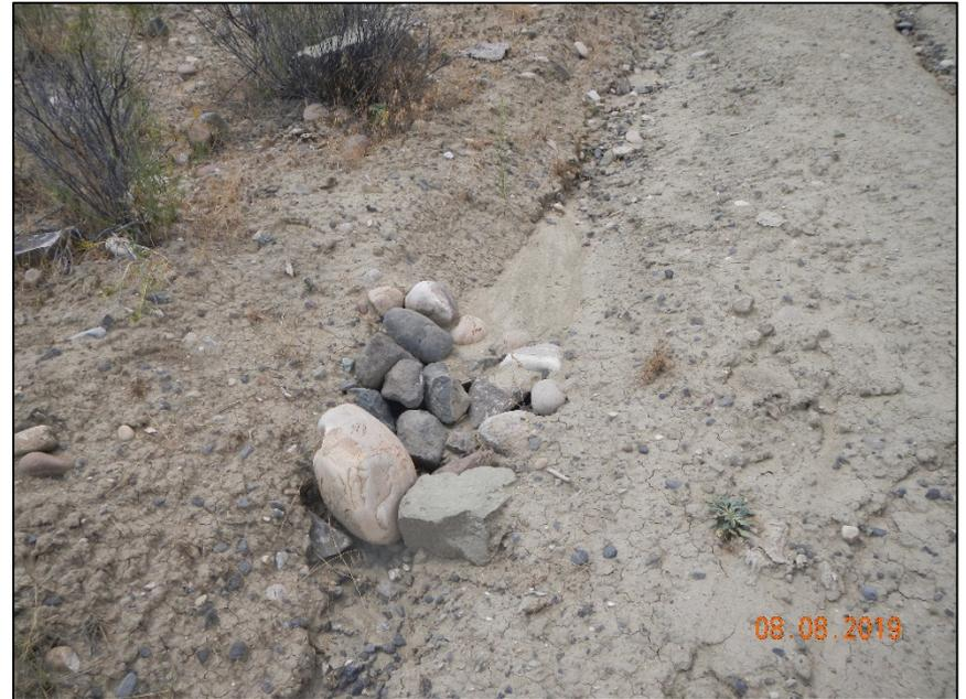
Photo #11 Check dams on access road need maintenance
