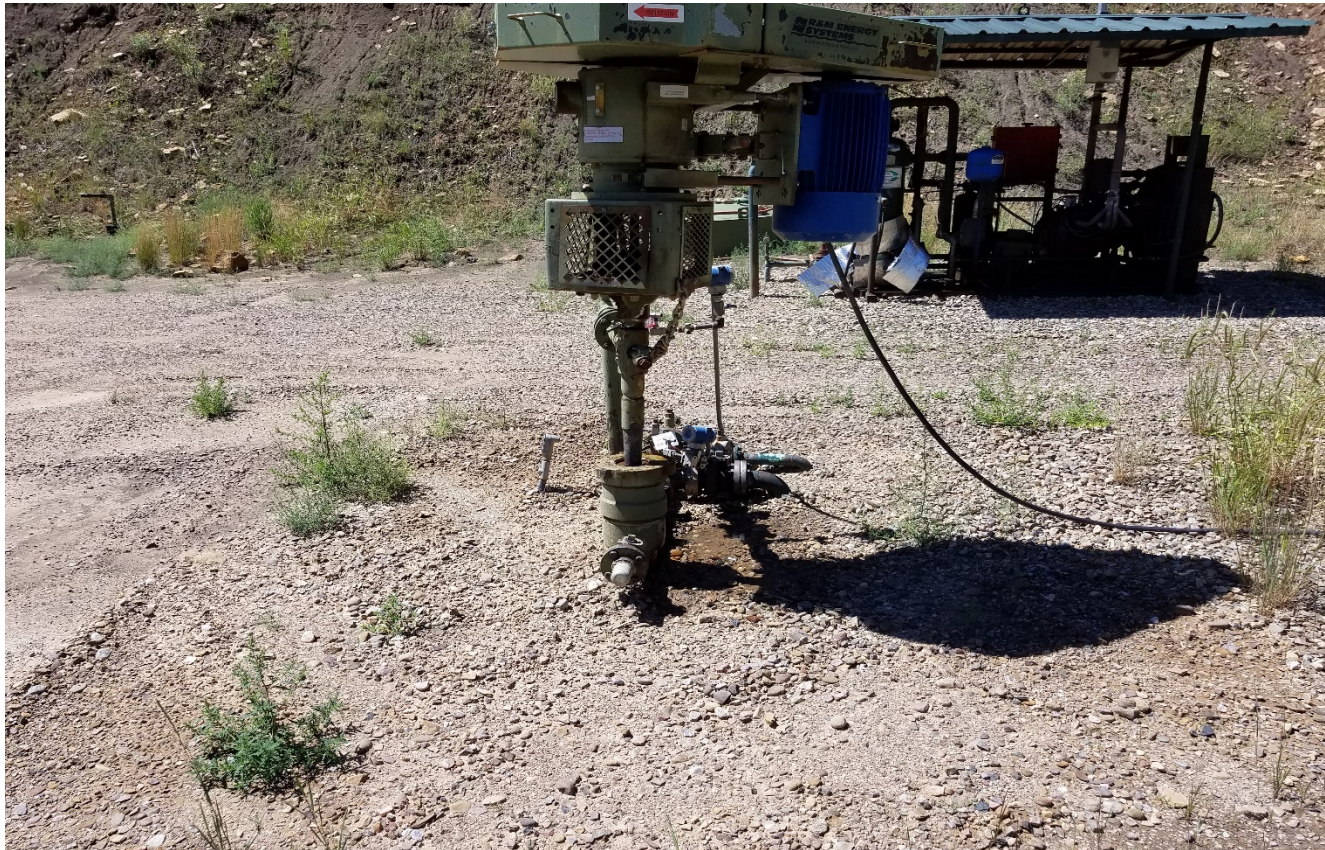
Photo 2. There is a dripping water leak from the wellhead.
