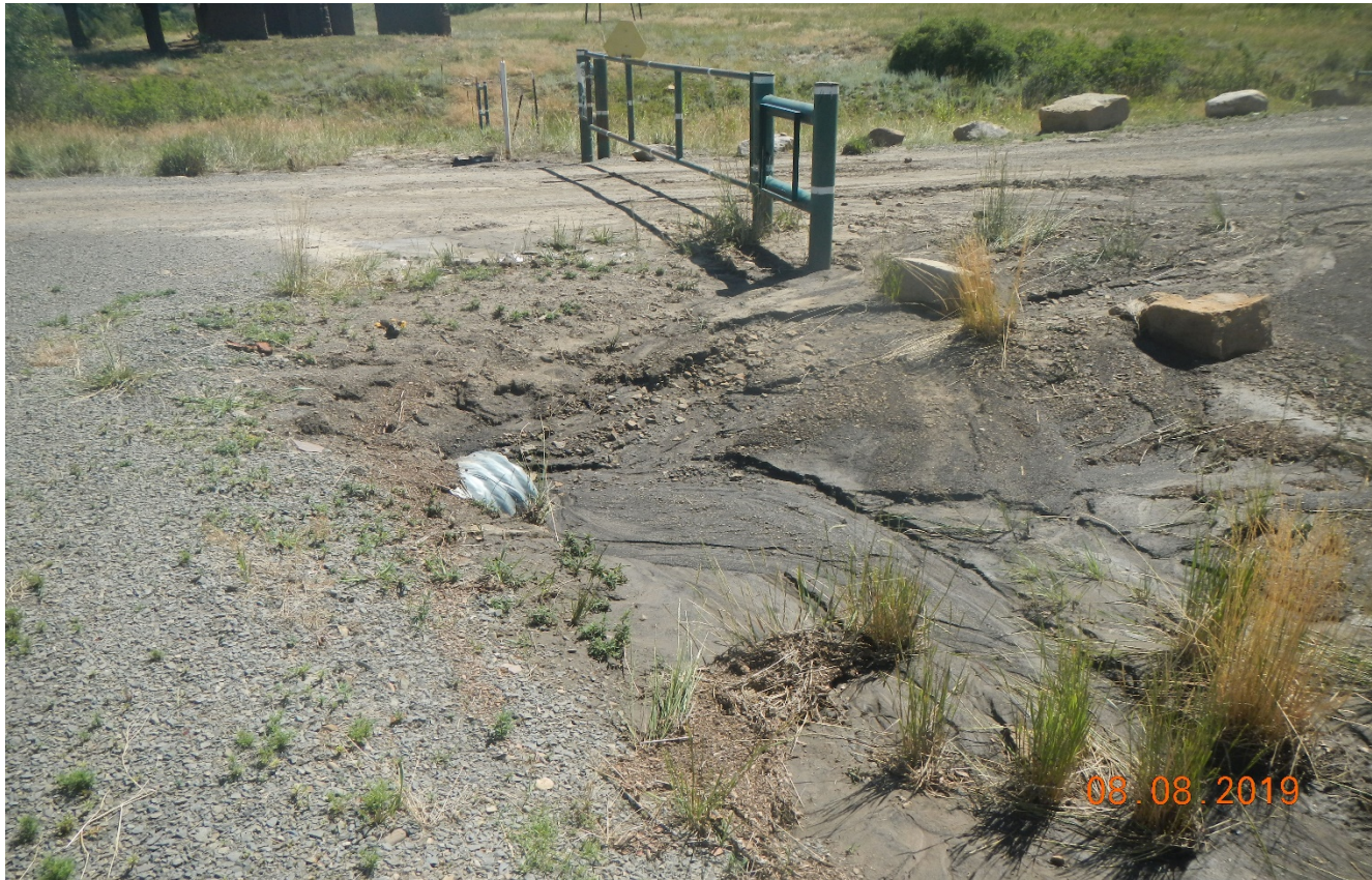
Photo 1. The culvert near the location has filled in with sediment. Erosion needs to be controlled from the source.
