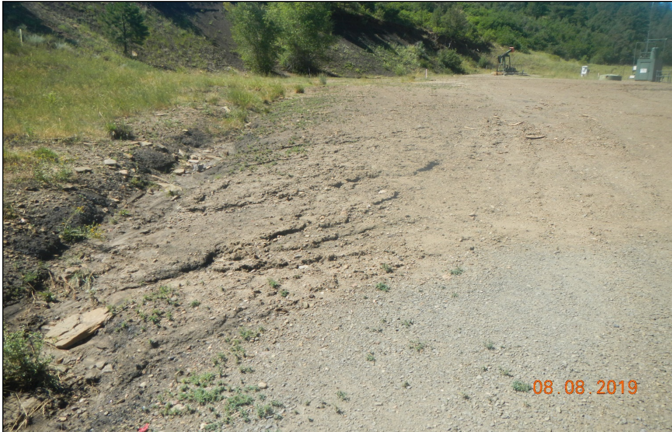
Photo 2. Erosion has been repaired however, this issue can occur again as rilling is beginning to occur.
