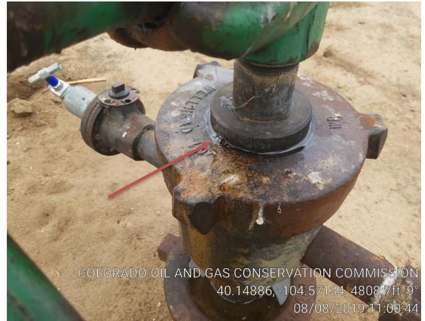
Pic 2 possible leak at wellhead
