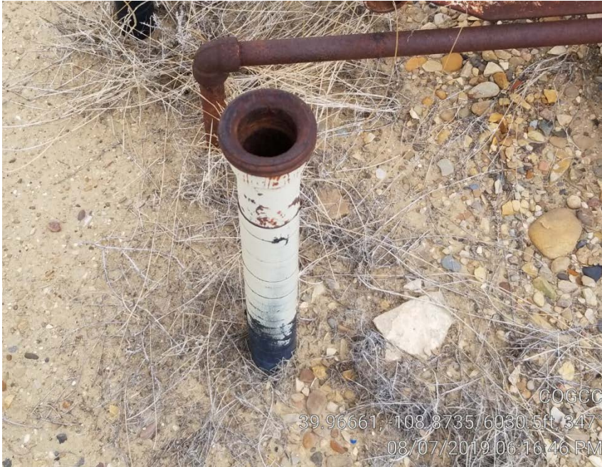
Photo 4. Uncapped riser next to separator.
