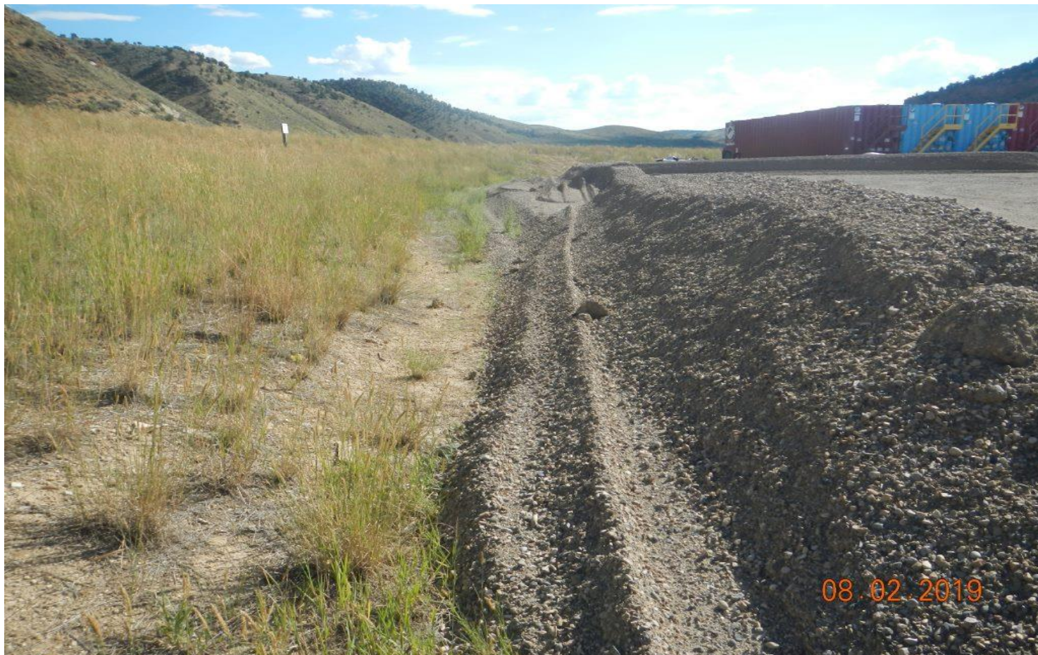
Photo#2: Berms constructed on East side of Pad.
