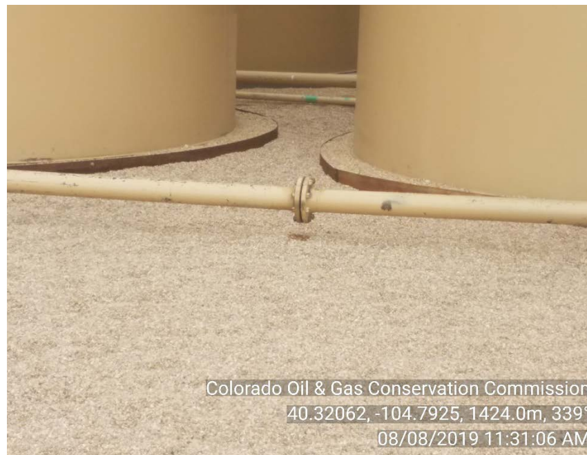
Photo #8 Load line leak
