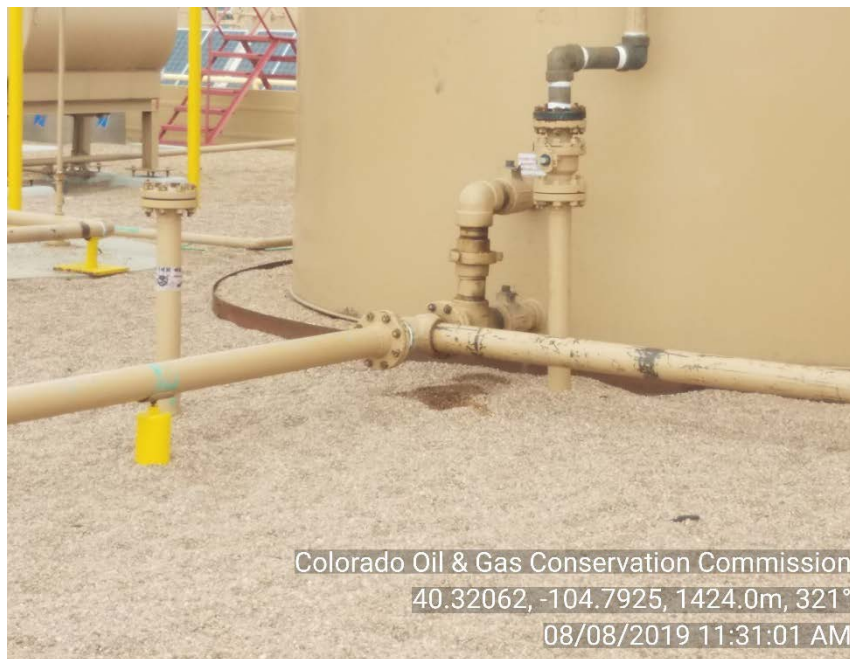
Photo #7 Load line leak
