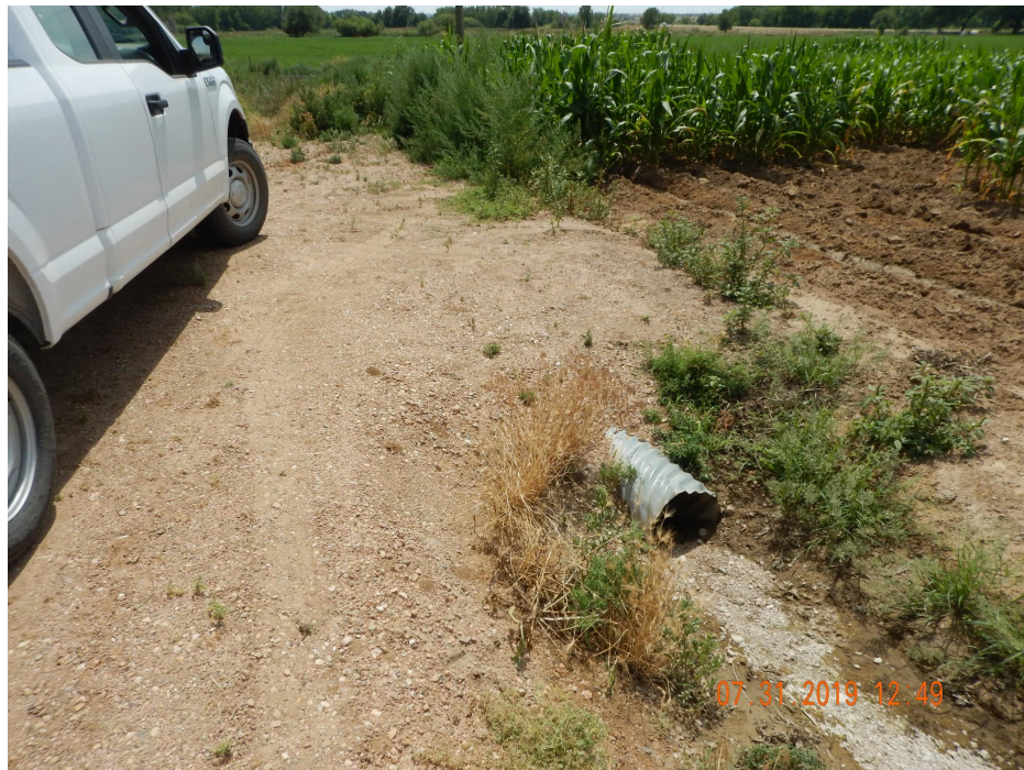
Photo 2. Photo taken from the south entrance to the tank battery location, facing South. Photo illustrates Operator has failed to remove the culvert.
