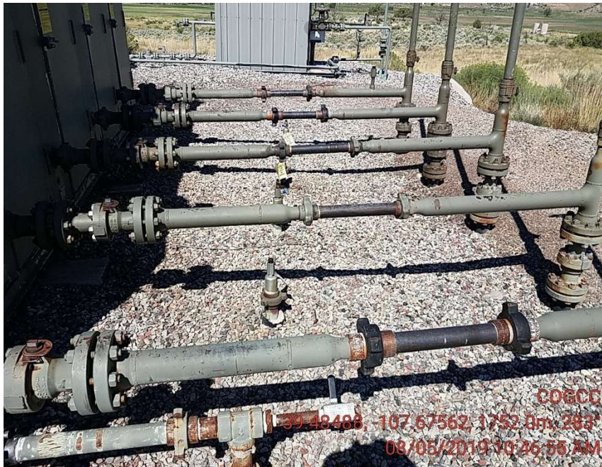
5 Disconnected lines tagged out
