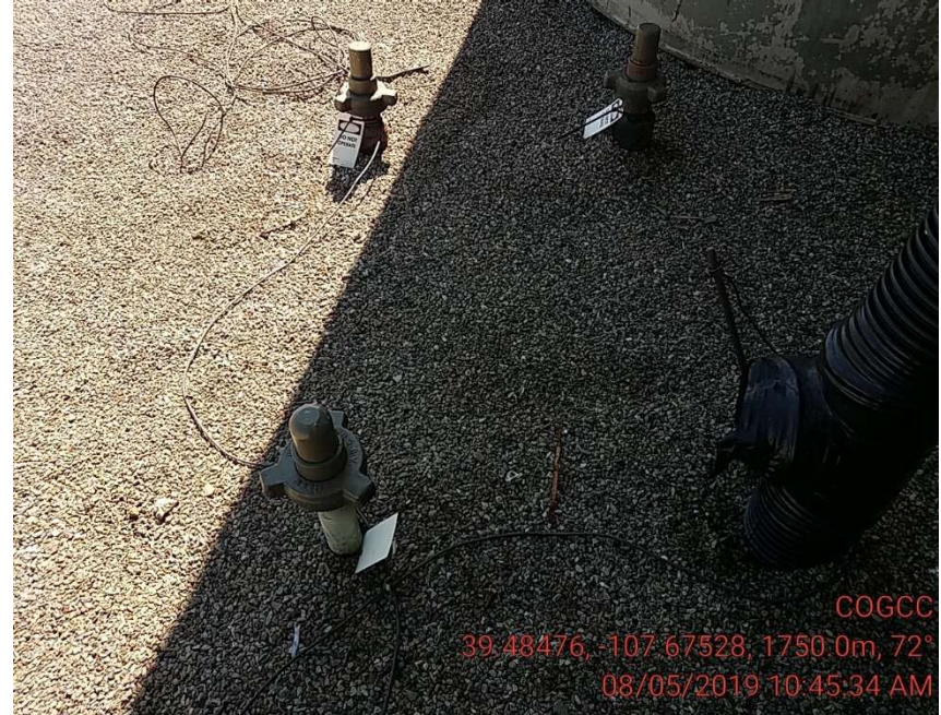
4 Disconnected lines tagged out
