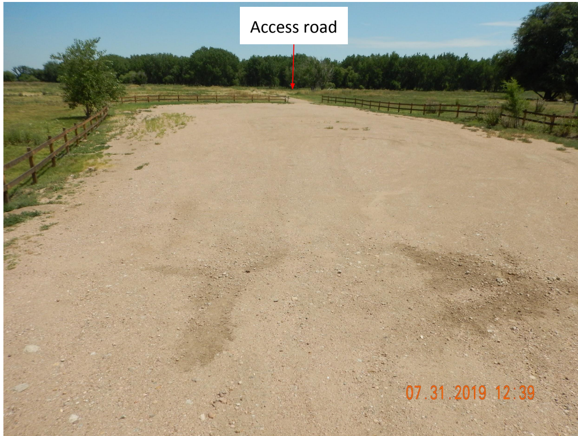
Photo 1. Photo taken from the entrance of the tank battery location, facing East. Photo illustrates the Operator has failed to reclaim the tank battery location and a portion of the access road to the well location. COGCC staff did not inspect the entire access road to the well location or the well location.
