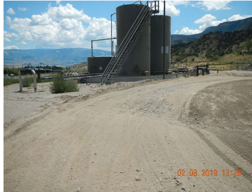
Photo #4 – Unlabeled 500 bbl ASTs. Ruts and erosions can also be seen.
