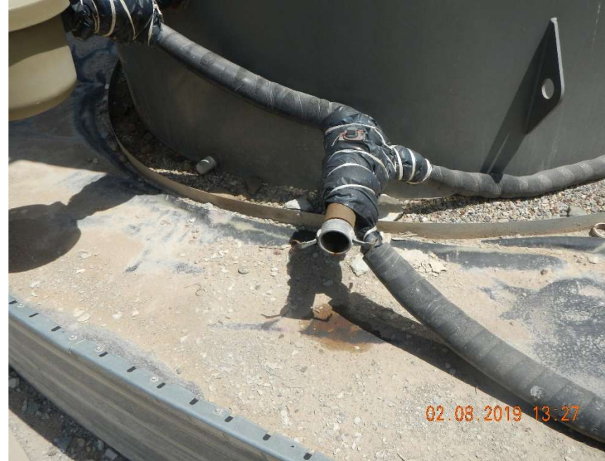
Photo #8 – Oil stained soil from 500 AST load out valve.
