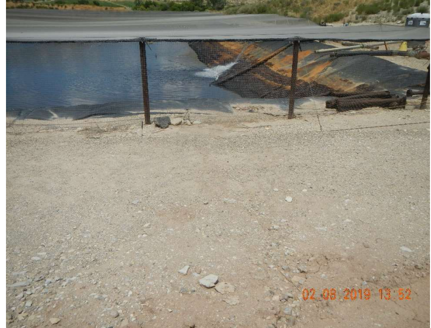
Photo #16 – Erosion leading into the south side of the pit.
