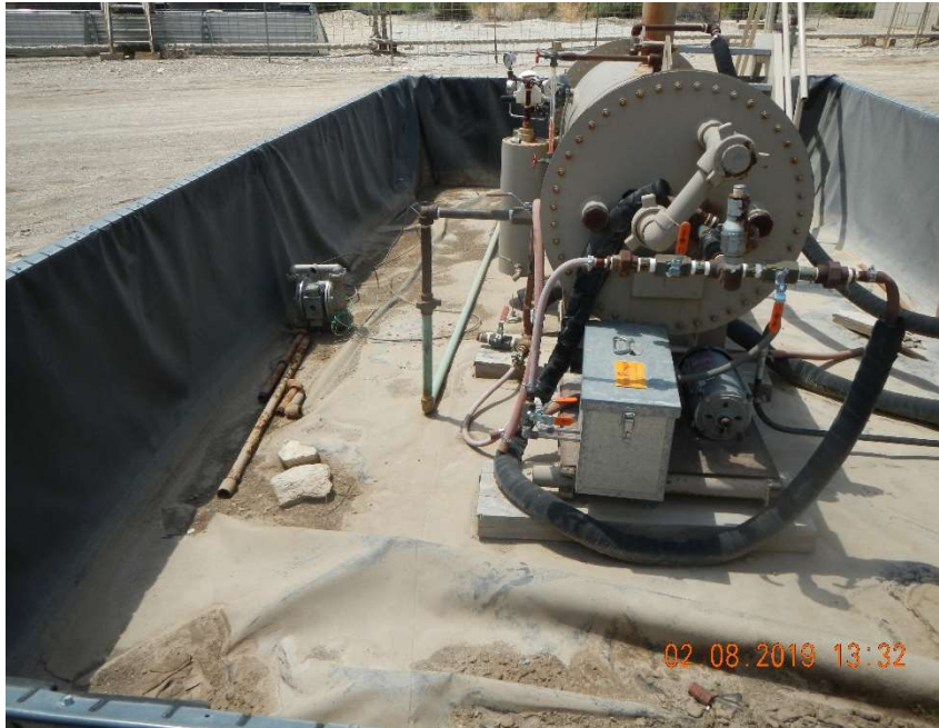
Photo #9 - Storage of equipment in separator secondary containment.
