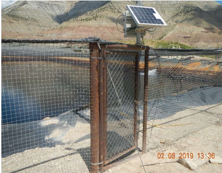
Photo #11 – Open gap in access gate located on the south side of the pit.
