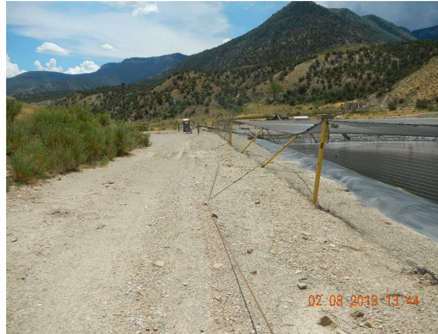
Photo #12 – Ballards on east side of the pit leaning to the west.
