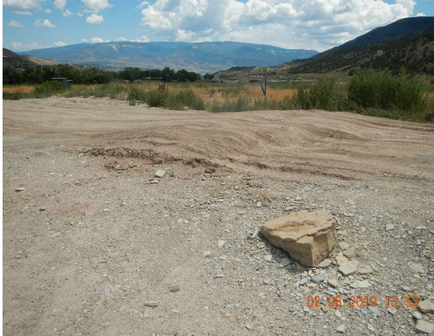
Photo #15 – Ruts and erosion on the south side of the pit.
