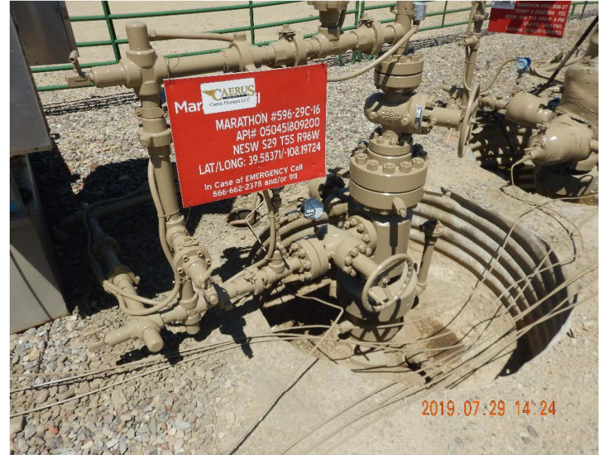
Photo #6 – Localized accumulation of oil-stained soil inside of Marathon 596-29C-16 cellar.
