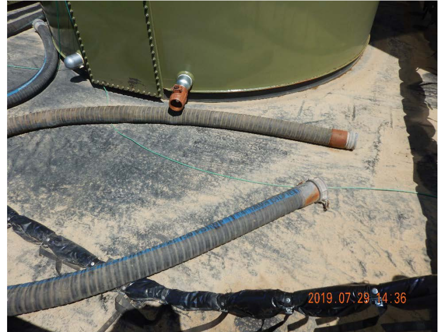
Photo #16 – Hoses stored inside of tank battery secondary containment with metal fittings in contact with liner.
