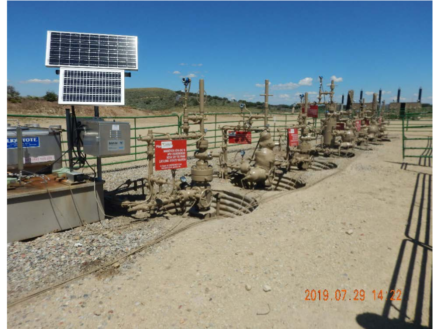
Photo #4 – View of wellheads, looking east. Note well cellars are uncovered.
