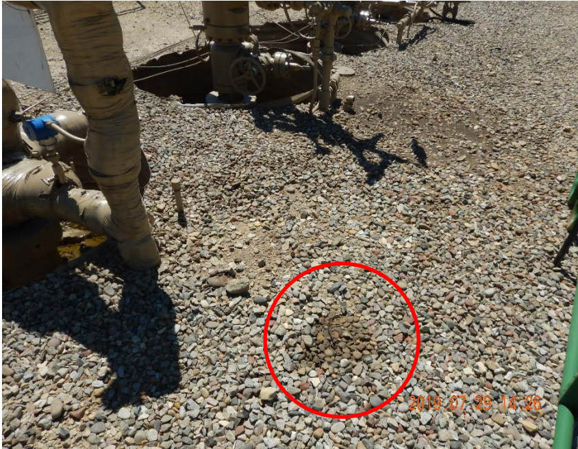
Photo #9 - Localized accumulation of oil-stained soil on north side of the Marathon 596-29C-25 wellhead.
