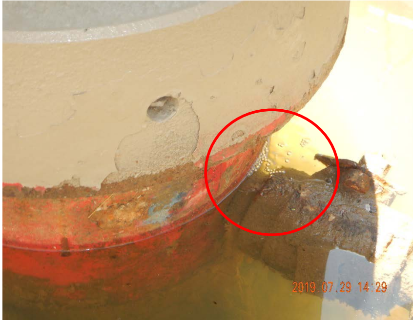
Photo #3 – Gas bubbling was observed from Marathon 596-29C-14 wellhead during inspection. Video is attached to this inspection report. Operator was notified via phone on inspection date.
