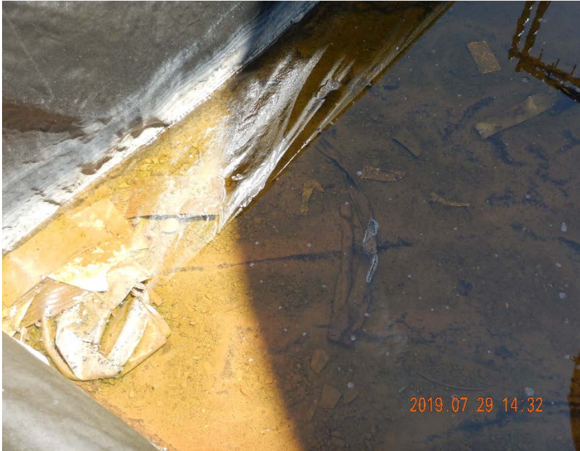
Photo #13 – Trash and fluid inside of tank battery secondary containment. No hydrocarbon sheens or odors were observed on fluids. No holes or tears were observed in visible portion of liner.
