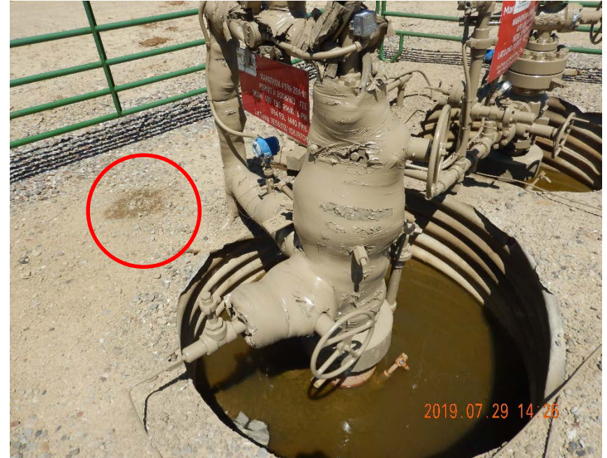
Photo #10 - Localized accumulation of oil-stained soil on north side of the Marathon 596-29C-18 wellhead.
