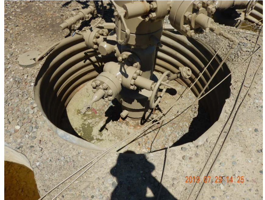
Photo #8 - Localized accumulation of oil-stained soil inside of Marathon 596-29C-12 cellar.
