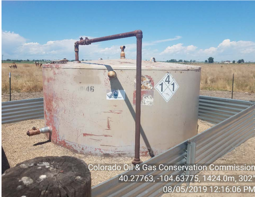
Gas sales tank placarding and berm
