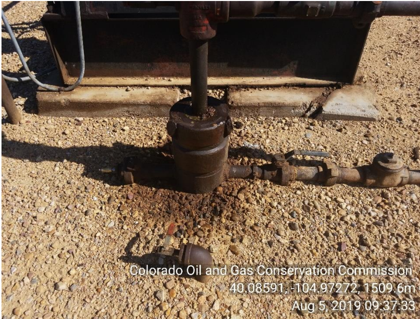
Photo 3 Stained soil around WH. Mechanical issue: appears packing is leaking.
