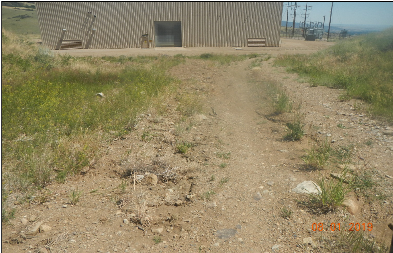
Photo 4. The area of erosion along the access road has been repaired. It is unclear if this area was reseeded for stabilization.
