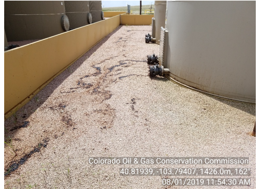
Photo #6 Horsetail 19N-1924M-R UIC - Disposal Facility Crude Oil Tanks - Drain lines Stained soil
