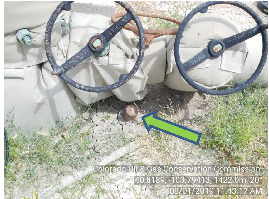
Photo #4 Horsetail 19N-1924M-R UIC - Wellsite Bradenhead Press: Bull plugged
