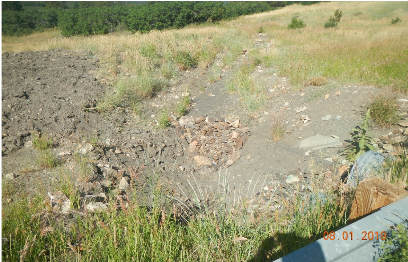
Photo 4. Sediment has been cleaned out of the culverts outlet. Material was placed off to the side which must be seeded and stabilized.
