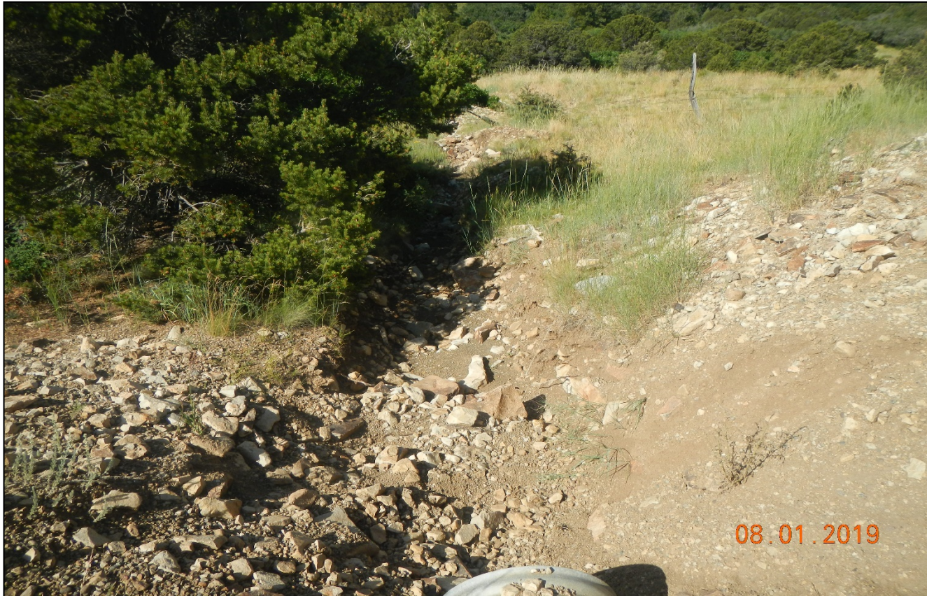
Photo 1. There is erosion occurring at the culvert with no outlet protection. No outlet protection has been installed at this culvert identified by previous inspection. Lat/Long:37.69799,-105.20237
