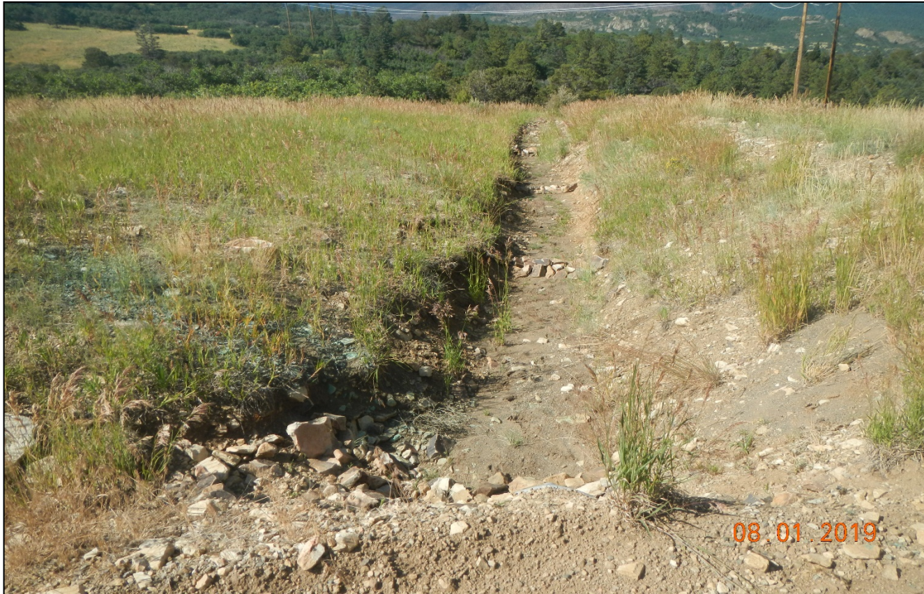
Photo 2. Rock check dams have been installed along the diversion ditch. These check dams are small and will likely fill in with sediment and will need ongoing maintenance. Lat/Long:37.69759,-105.201516
