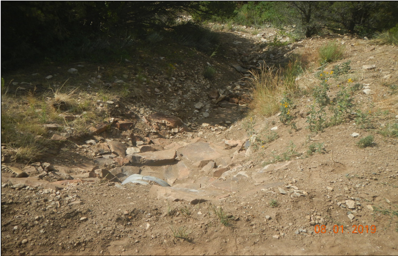
Photo 1. Rock rip/rap and check dams have been installed at the culvert outlet. Lat/Long:37.69957,-105.22668
