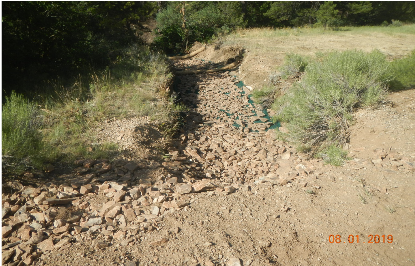
Photo 3. Erosion channel has been repaired at the culvert outlet. Rock rip/rap, wattles, and erosion matting was placed in channel. It is uncertain if rip/rap is large enough to handle high water flow in heavy rain events.
