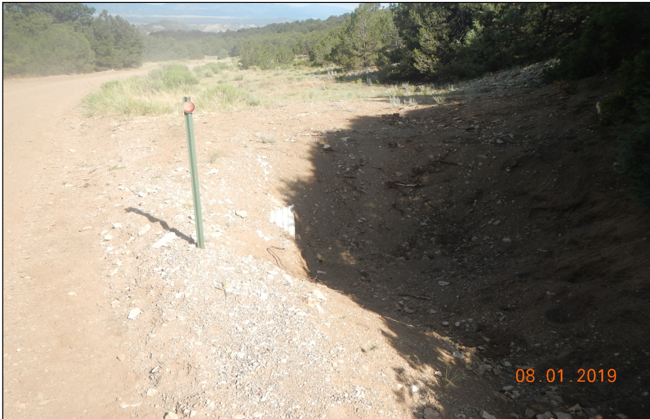
Photo 2. Sediment at culvert inlet has been removed.
