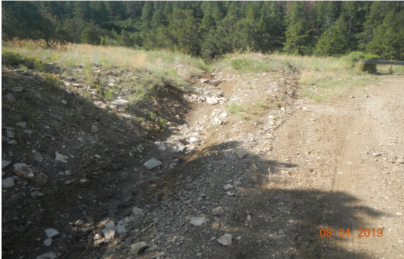
Photo 4. Rock check dams have been installed along the diversion ditch. These check dams are small and will likely fill in with sediment and will need ongoing maintenance. Lat/Long:37.69860,-105.21673
