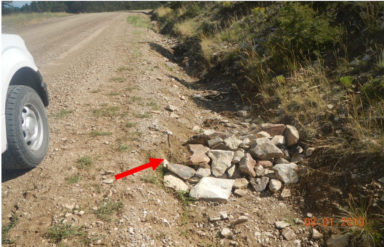
Photo 5. Rock check dams have been installed along the side of the road. The low point of the check dams should be in the center and on this one it is on the side shown by arrow. Stormwater will flow toward the side and will erode the into road. Lat/Long:37.69860,-105.21673
