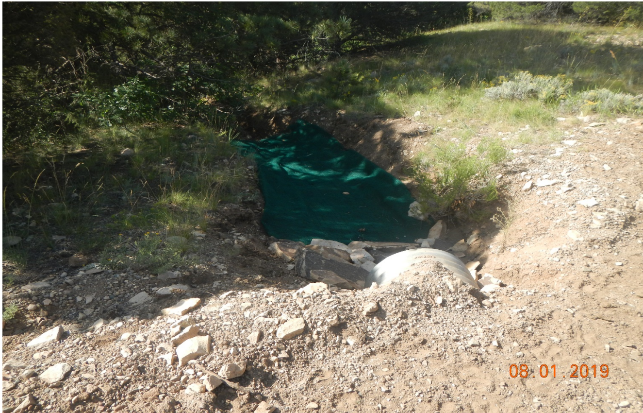
Photo 6. Erosion channel has been repaired at the culvert outlet. Rock rip/rap and erosion matting was placed in channel. The matting is not trenched in on the side and could become displaced.
