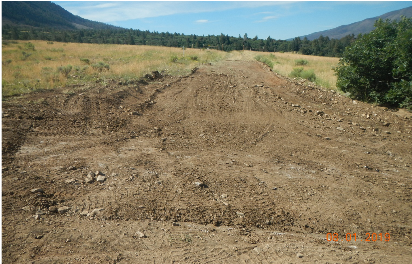
Photo 7. Facing south toward the access road. Which was graded. This area needs to be stabilized.
