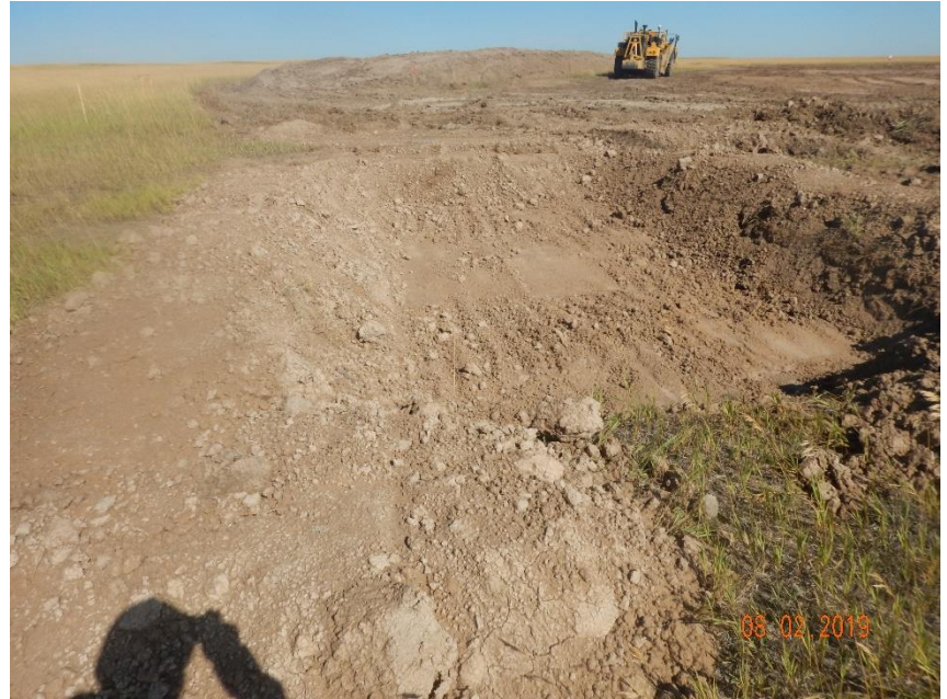
Photo 6: Photo taken from the south end of the location, facing west. Photo shows 1 of the 3 sediment traps constructed on the south end of the location. BMPs have not been constructed in accordance with good engineering practices; berms along perimeter have not been sufficiently consolidated, trap has not been constructed at an appropriate grade to mitigate stormwater degradation, BMP missing sufficient inlet and outlet protection.
