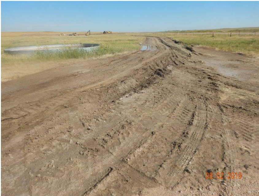
Photo 13: Photo taken from the access road, facing north. Road currently wet/muddy due to recent rain event. Vehicle tracking BMPs missing from access road. Additionally, access road appears to have been constructed across, and damming, a drainage. No BMPs (such as a culvert) has been installed to allow stormwater movement. Access road does not appear to have been constructed in such a manner to mitigate degradation or sediment transport per 1002.f and 1002.e.
