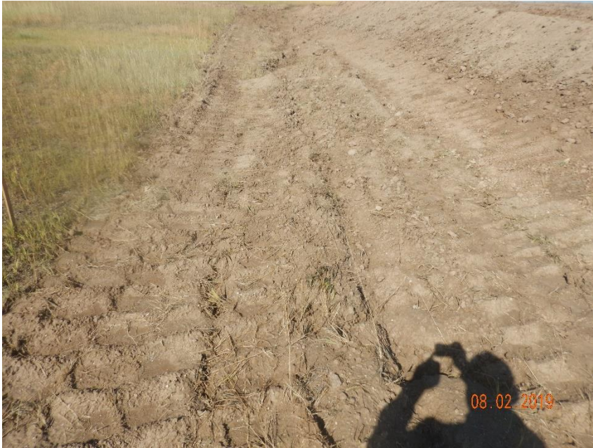
Photo 5: Photo taken from the south end of the location. Photo shows operator has installed surface roughening (ripping) along perimeter of the disturbance. Surface roughening is a temporary BMP that needs to be used on conjunction with other BMPs. Surface roughening on the southern perimeter of the location appears to have been traveled over and is not longer in proper functioning condition.
