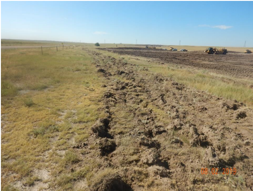
Photo 9: Photo taken from the east end of the location facing south. Photo of surface roughening BMP
