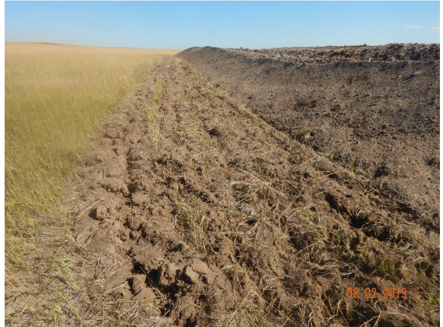
Photo 8: Photo taken from the west end of the location, facing north. Photo shows surface roughening BMP on the western perimeter of the location. Photo also shows soil stockpiles. Soil stockpiles have not been stabilized or BMPs installed in accordance with 1002.c
