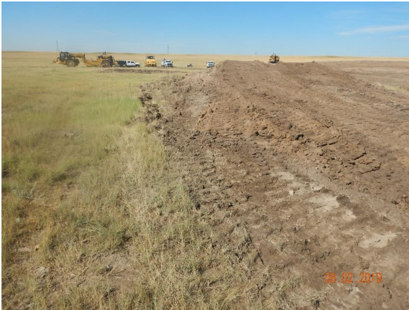
Photo 11: Photo taken from the southeast corner of the location, facing west. Photo shows areas of surface roughening on the southern perimeter that have been traveled over and is no longer in proper functioning condition
