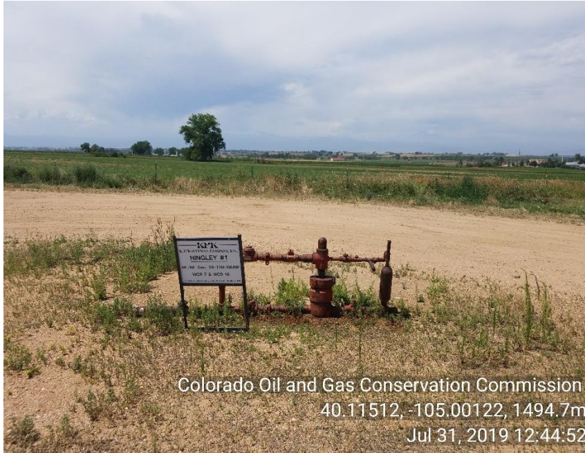
Photo 1 WH sign and stained soil around WH
