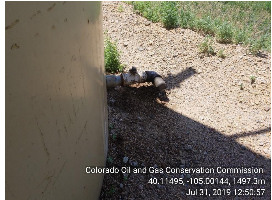
Photo 14 stained soil under Produced water tank load line.
