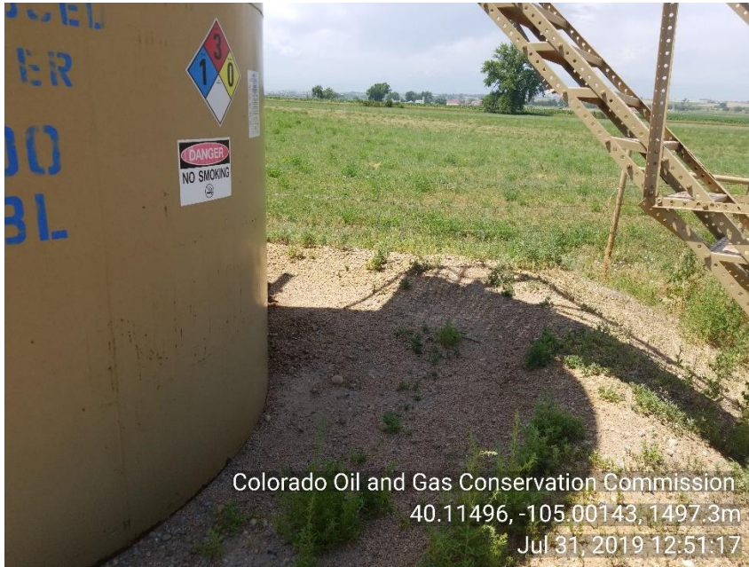
Photo 15 Inadequate berms around produced water tank.
