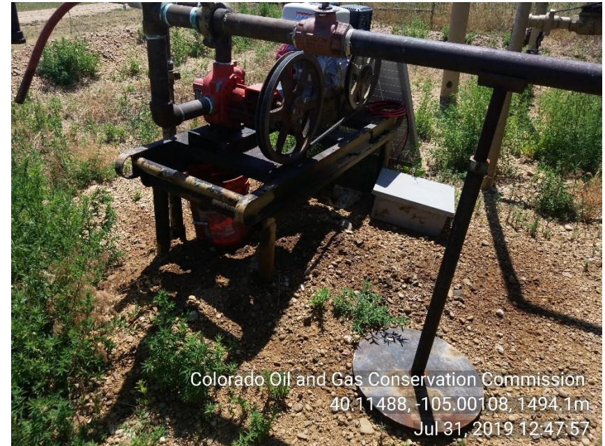
Photo 8 Stained soil around re circ pump. Mechanical issue: re circ pump.
