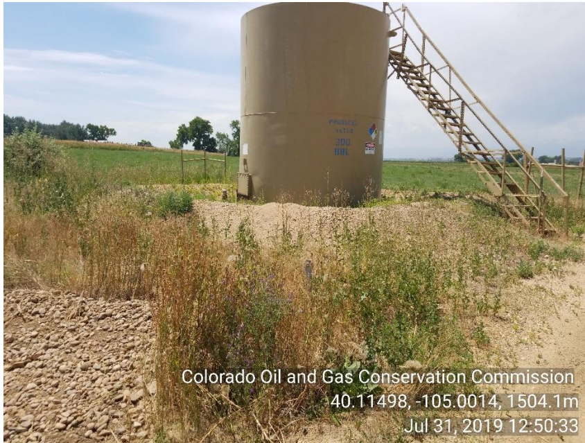
Photo 13 Produced water tank. Weed in and around containment.
