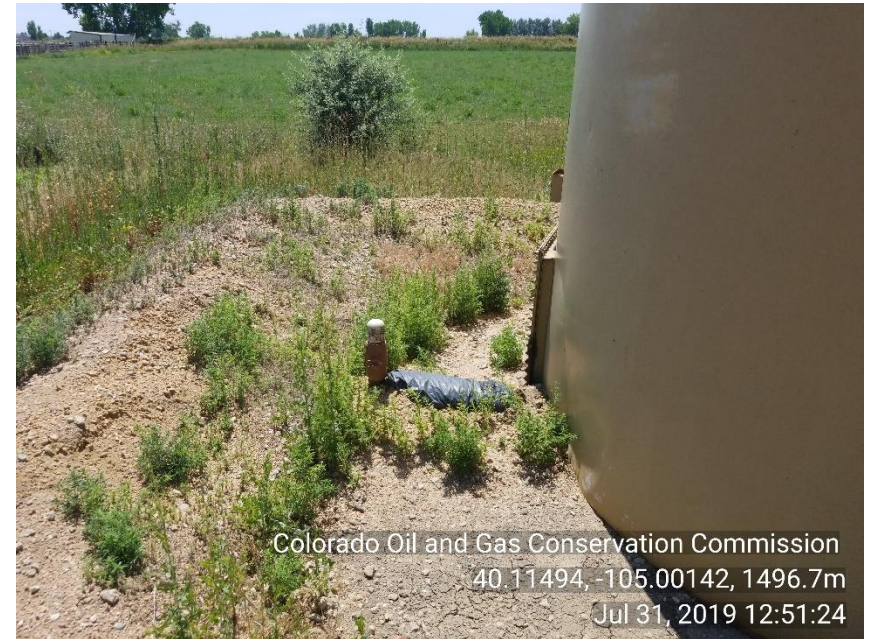
Photo 16 Inadequate berms around produced water tank.
