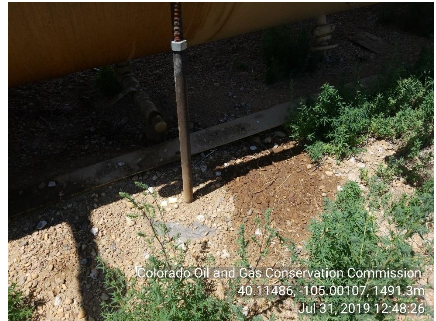
Photo 10 Stained soil under and around HOZ SEP
