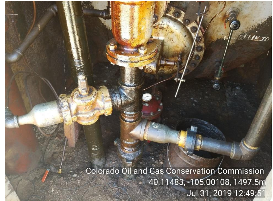
Photo 12 Mechanical issue: Piping visibly appear to be covered in what appears to be Produced fluid. Stained soil underneath piping of HOZ SEP.
