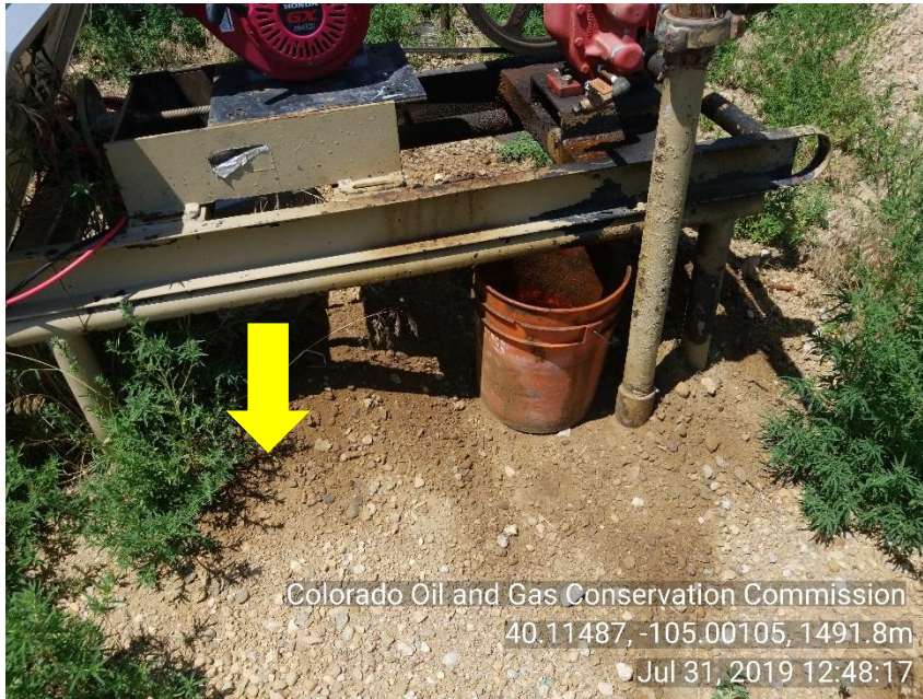
Photo 9 Stained soil around re circ pump. Mechanical issue: re circ pump.
