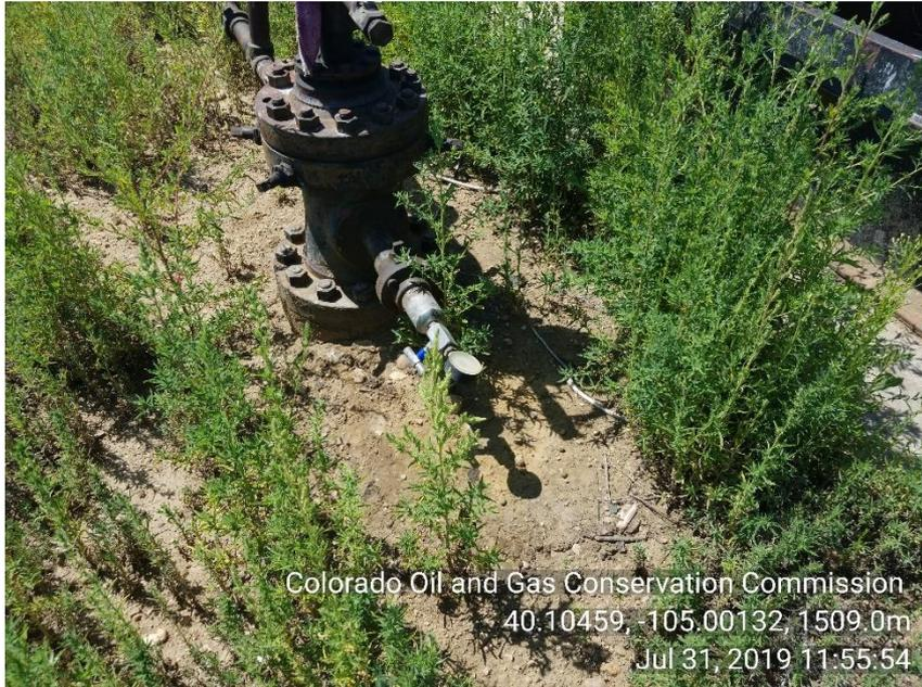
**Photo 3 Stained soil around well head. Weeds around WH.**
