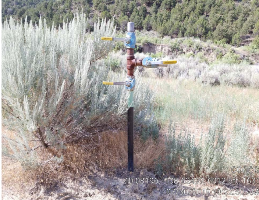
Photo 3. Gas line riser.
