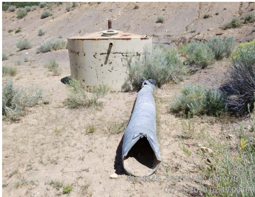
Photo 10. Damaged culvert.
