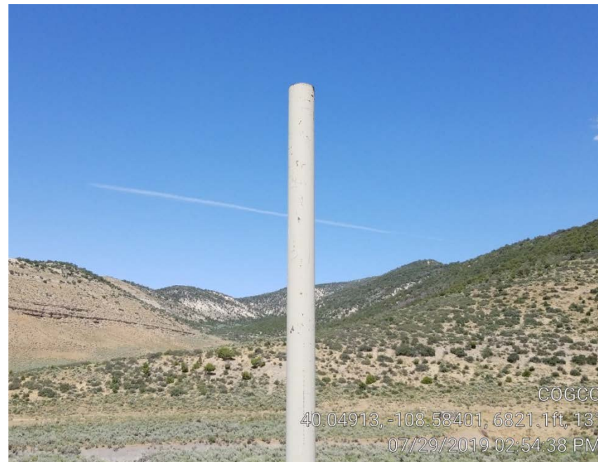
Photo 7. No apparent bird screen on tank vent.
