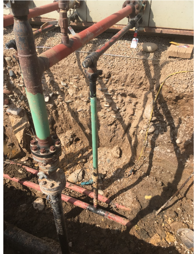
2" Dump line, leak discovered at tee
