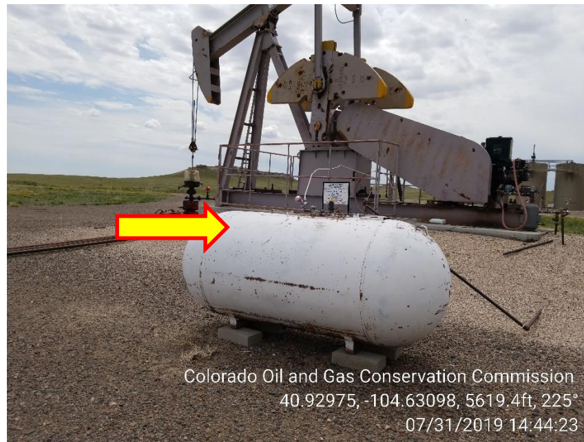
Photo 2 – Propane Tank, missing labels.
