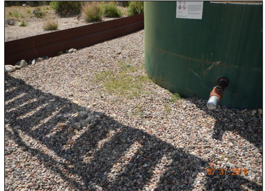
**Photo #5 Weeds growing inside of tank containment**
