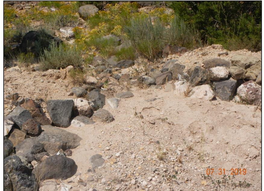
**Photo #10. Sediment trap on the west side of location, that all secondary perimeter ditches feed into, is in need of maintenance.**
