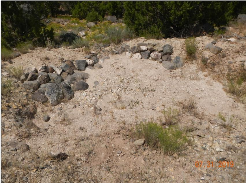
**Photo #9. Sediment trap on the west side of location, that all secondary perimeter ditches feed into, is in need of maintenance.**
