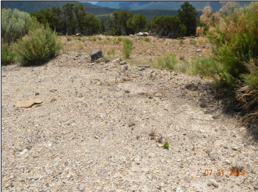
**Photo #7 Berm around location is used as a BMP and needs maintenance and made to meet COGCC specifications**
