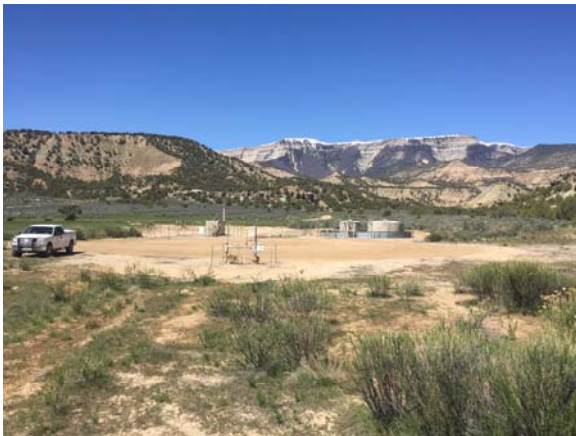
PAD OVERALL LOOKING WESTERLY
