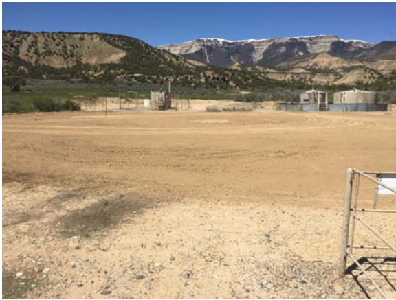
PAD LOCATION LOOKING WEST
