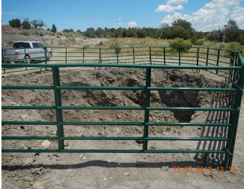
Photo #3 – View of the pit excavation looking east.
