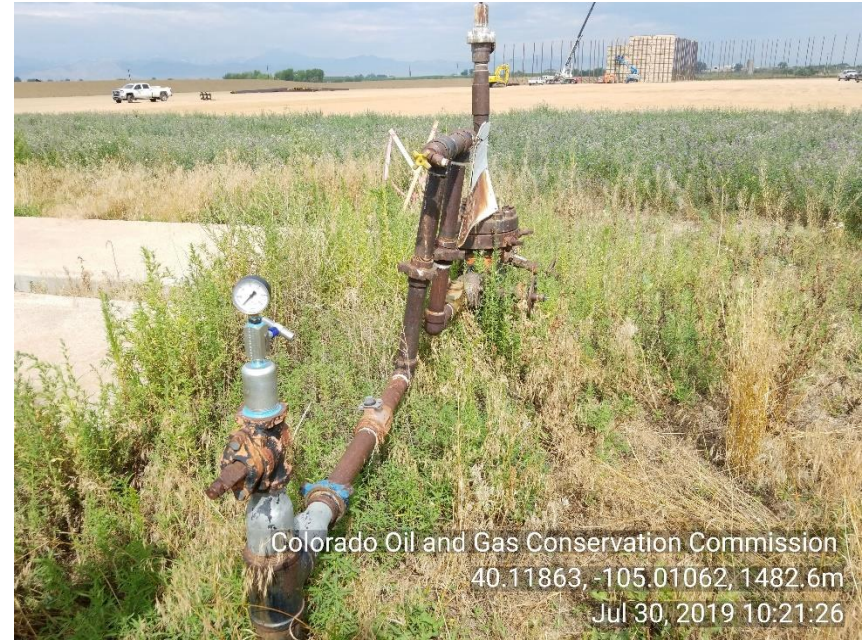
Photo 4 Weeds around WH. 2" flow line appears to be closed well is shut in.
