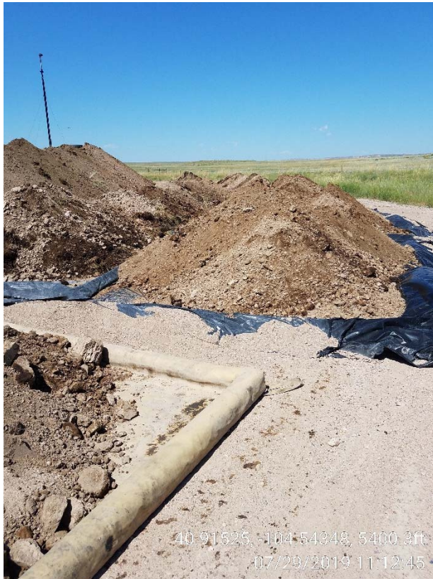
Photo 9 – Stockpiles of impacted material placed on liner.
