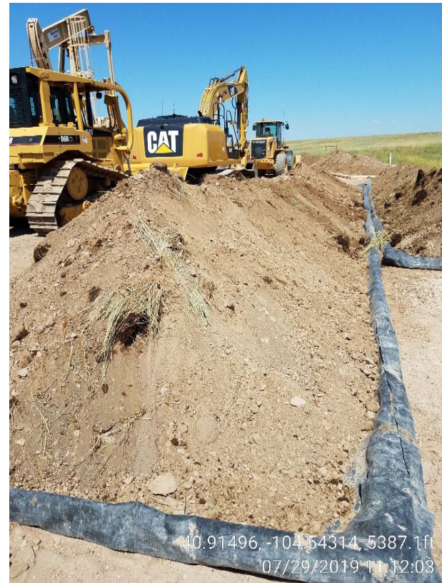
Photo 8 - Stockpiles of impacted material placed on liner.
