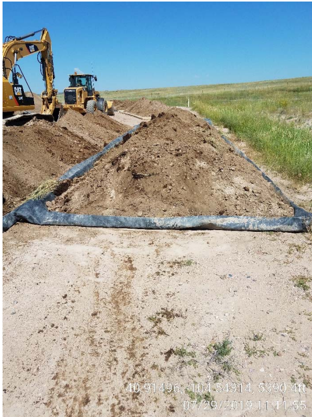
Photo 7 – Stockpiles of impacted material placed on liner.
