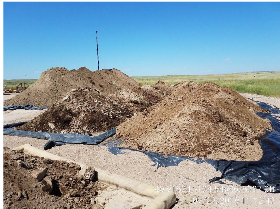
Photo 10 - Stockpiles of impacted material placed on liner.
