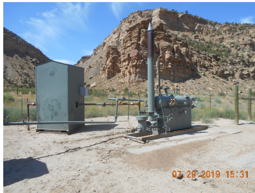
Separator and Meter housings. Junk pipe removed. CA completed.
