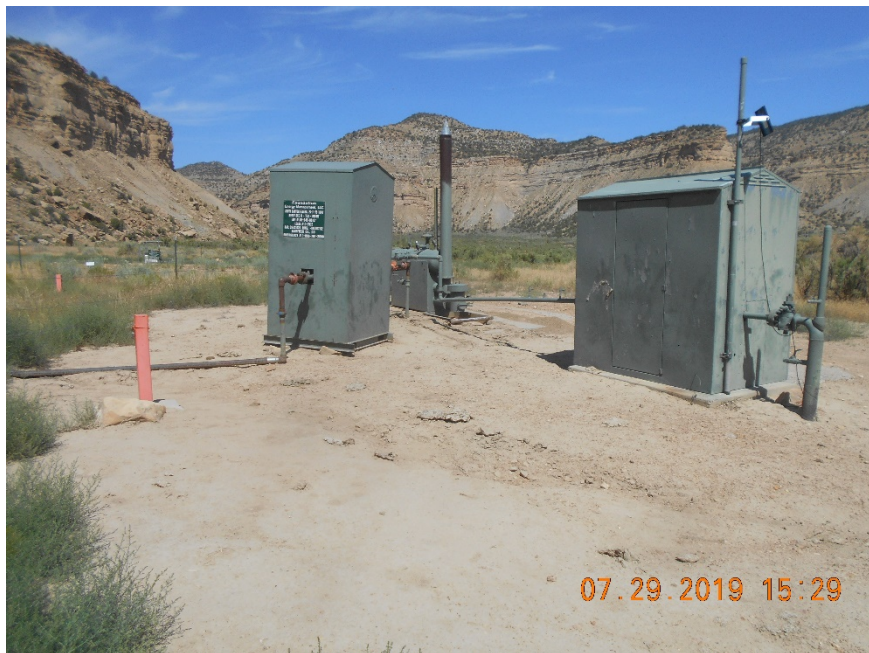
Separator and Meter housings.
