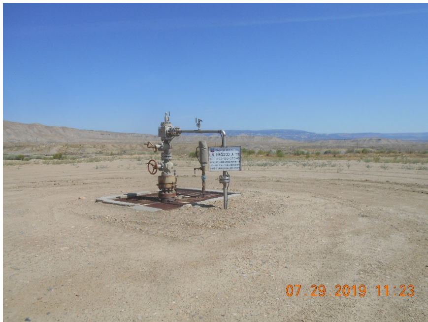
Injection wellhead with sign.
