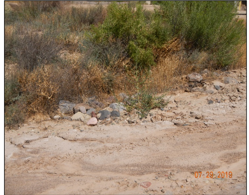
Photo # 16 BMP on SW corner of entrance to location needs maintenance. Sediment moving off location and down access road.
