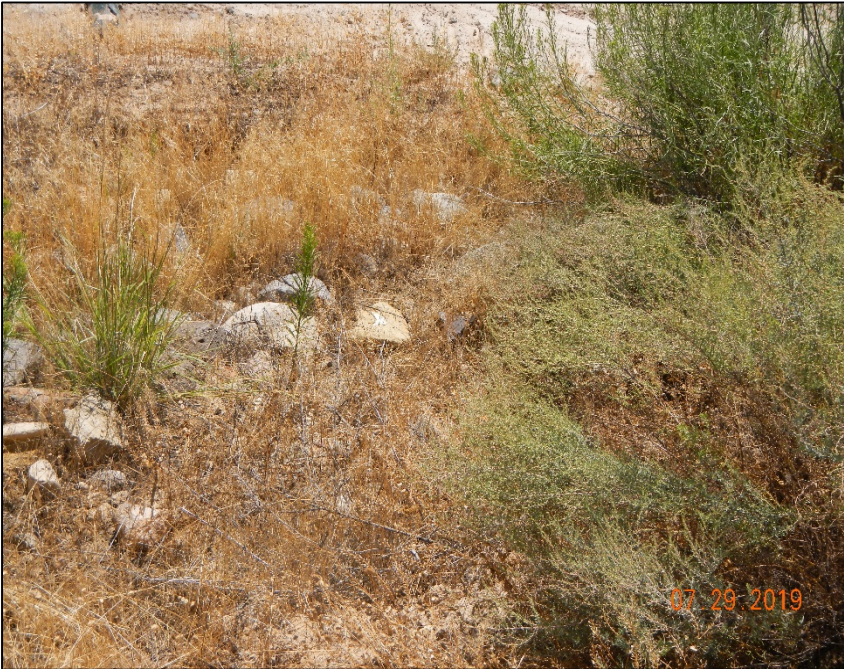
Photo # 15 BMP on SW corner of entrance to location needs maintenance. Sediment moving off location and down access road.
