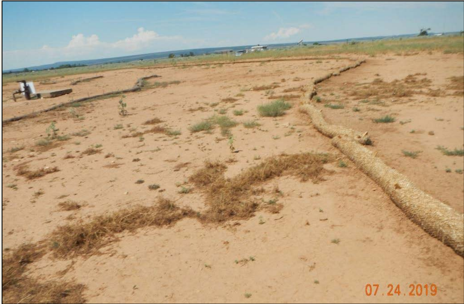
Photo 1. View of perimeter wattle in the northern project area facing westward.
