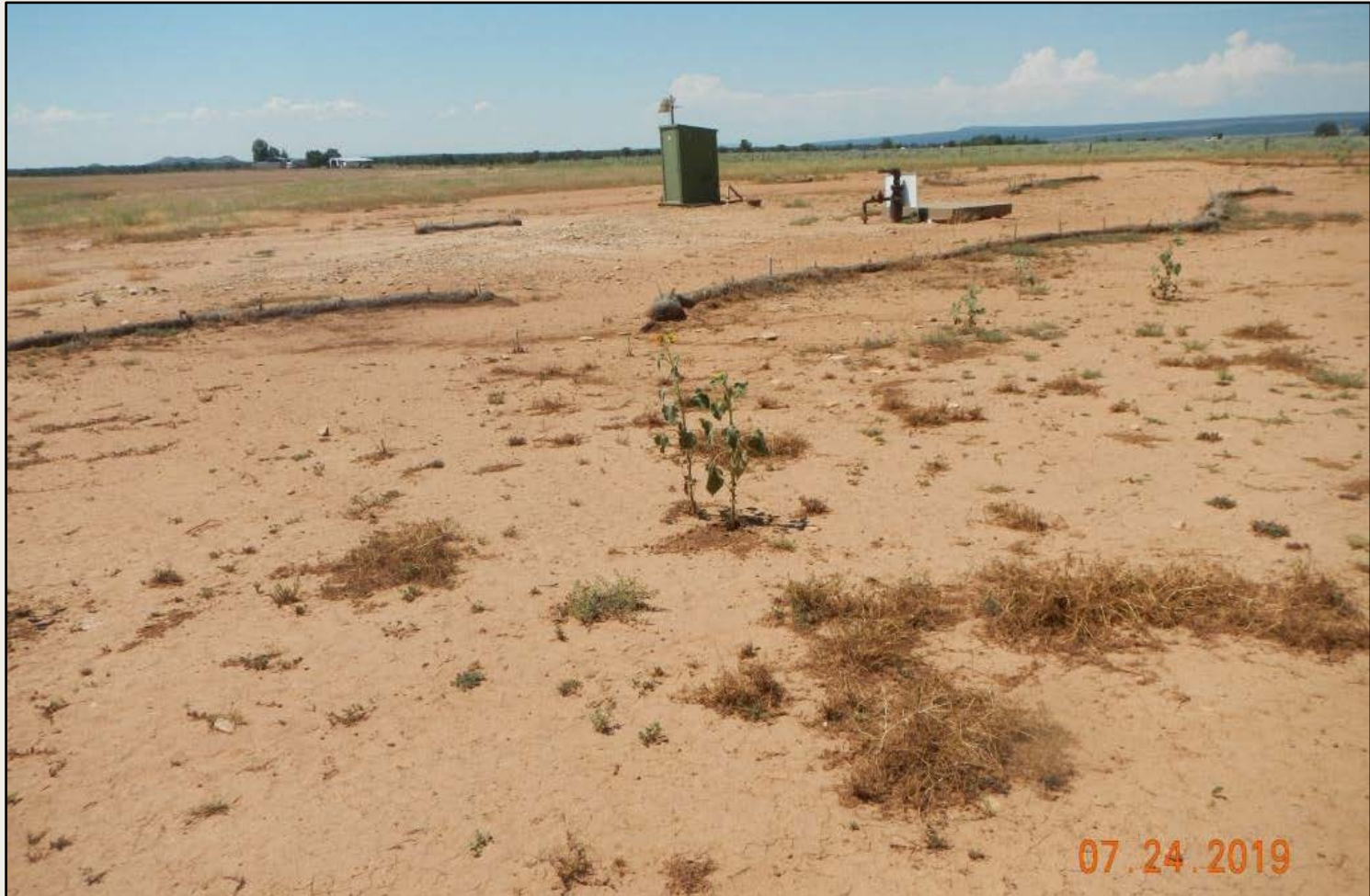
Photo 2. View of project area from the northern edge facing center. Wattles are largely functioning. Minor new erosion observed where wattles are not sufficient to de-energize surface flows.
