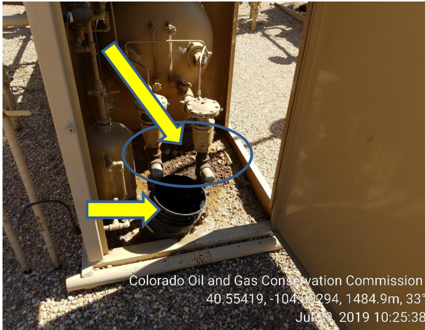
Photo 9: Stained soil (middle) separator/bucket with unknown contents
