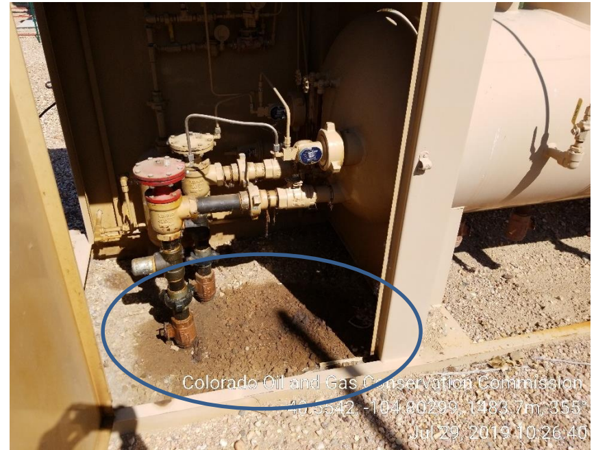
Photo 10: Stained soil (W) separator
