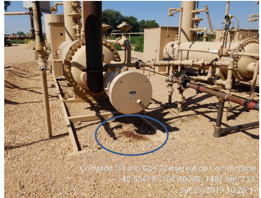
Photo 12: Stained soil (E) separator
