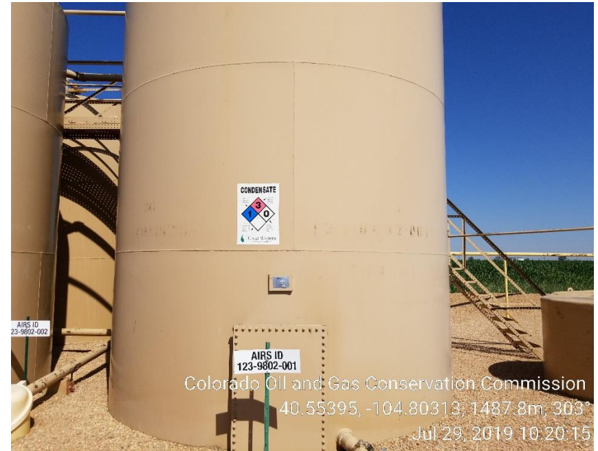
Photo 2: (North) Condensate tank with no labeling
