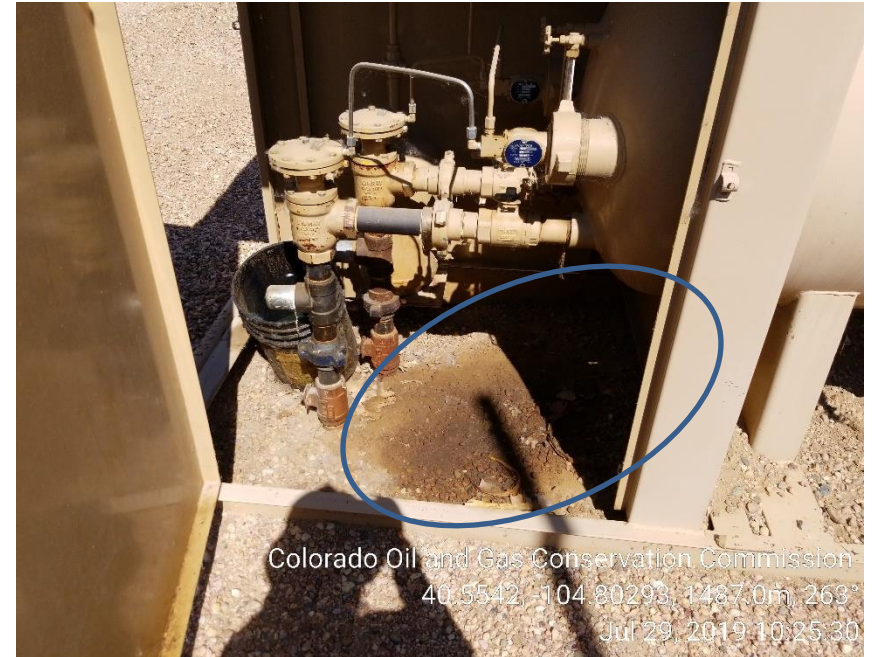
Photo 8: Stained soil (middle) separator
