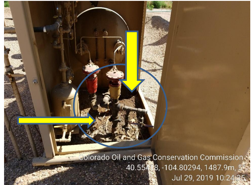
Photo 6: Stained soil (E) separator
