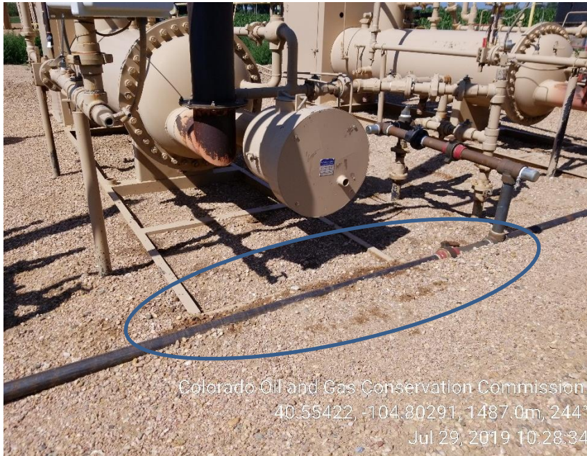
Photo 13: Stained soil (middle) separator
