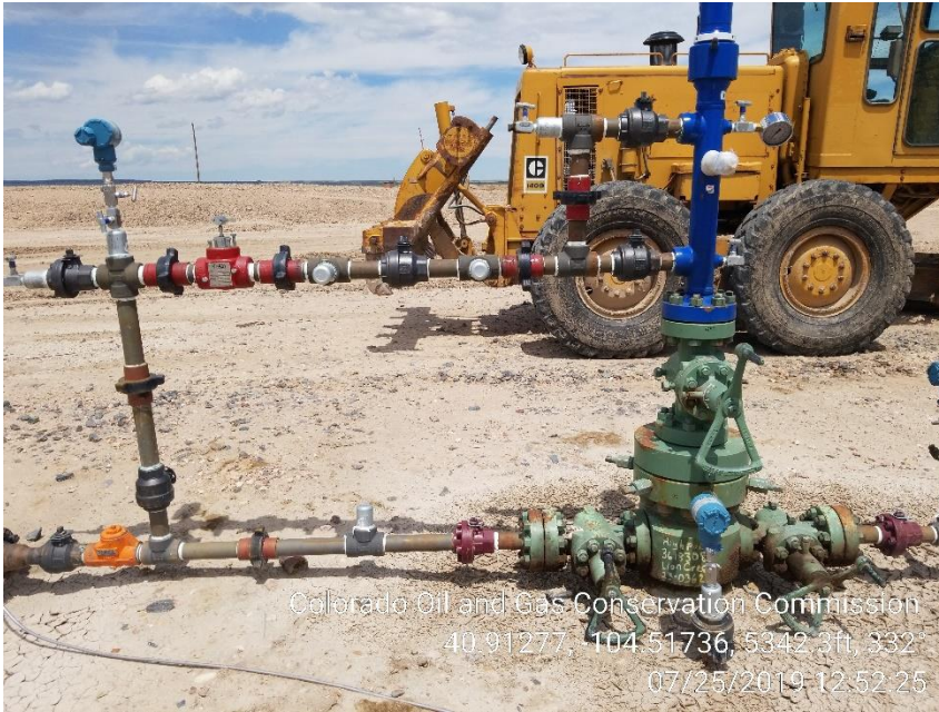
Photo 7 – West Wellhead, labeled Lion Creek 23-0362B, missing Wellhead sign
