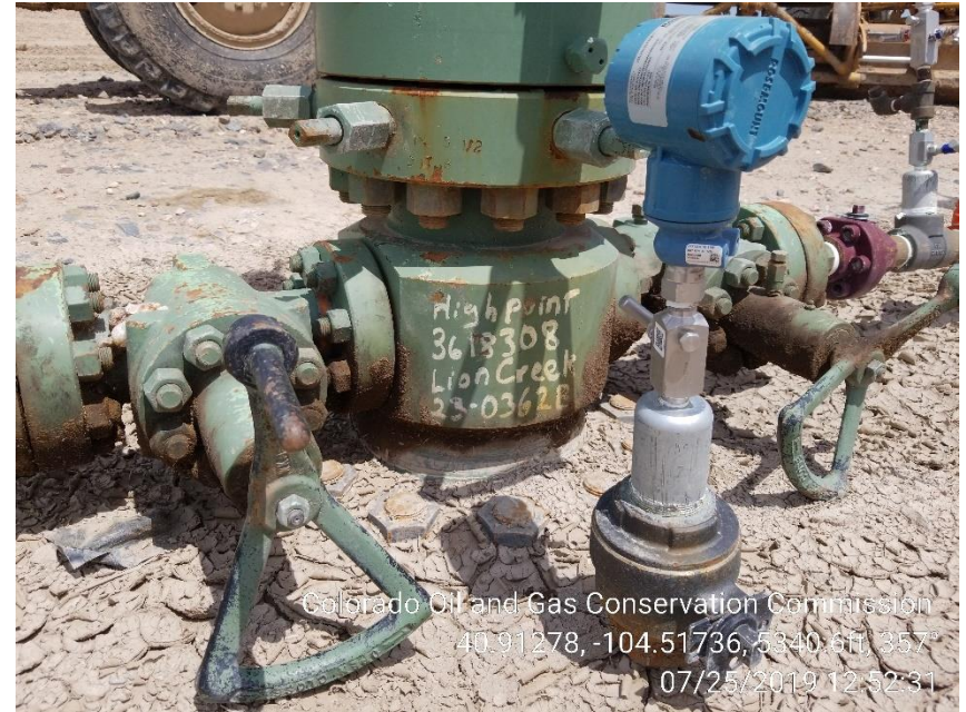
Photo 8 – Middle Wellhead, labeled Lion Creek 23-0362B
